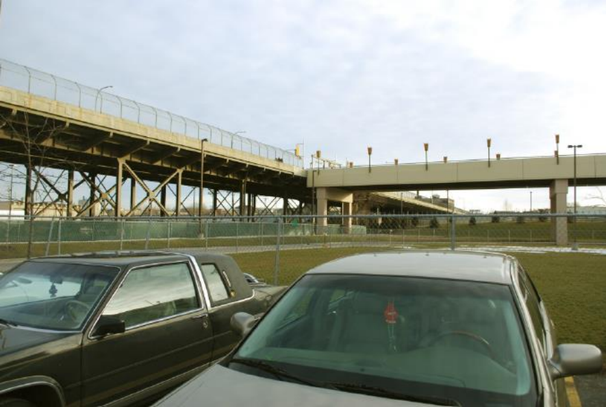
Southeast view from site
