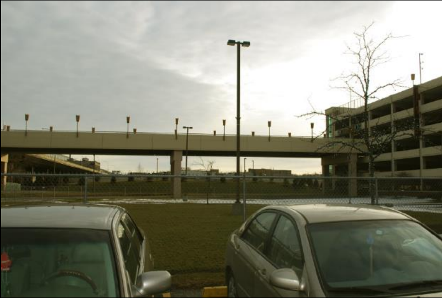
South view from site
