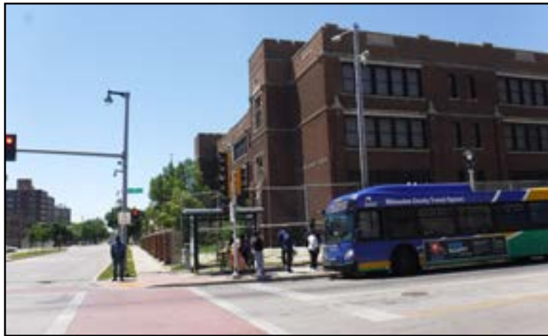
The former Wisconsin Avenue School at the northwest corner of North 27th and Wisconsin Avenue.
