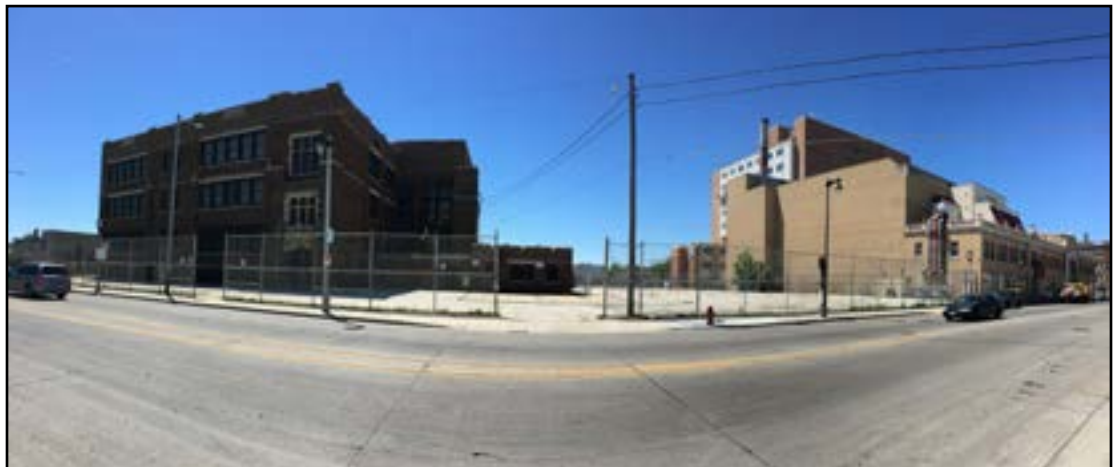
Current conditions on the Wisconsin Avenue School grounds.
