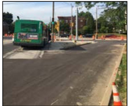
Right turn bypass lane at the intersection of North 27th and Highland Avenue.
