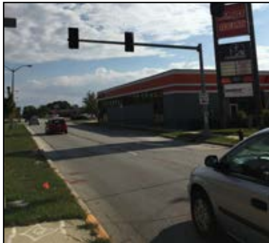
A more ideal monotube design used at South 60th and West Forest Home Avenue.
