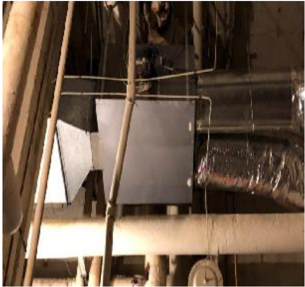
Figure 16: Original dual duct box
