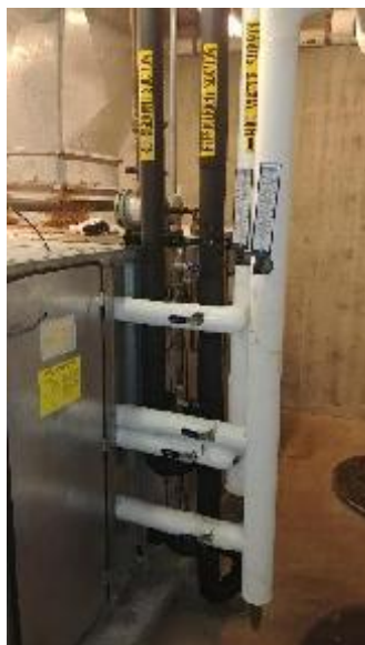
Figure 29: AHU-1 DX coil connections
