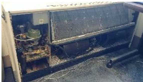
Figure 22: Existing Fan Coil unit (Interior)
