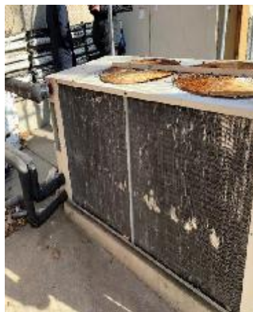
Figure 38: ACCU-2 outdoor unit, with rust.
