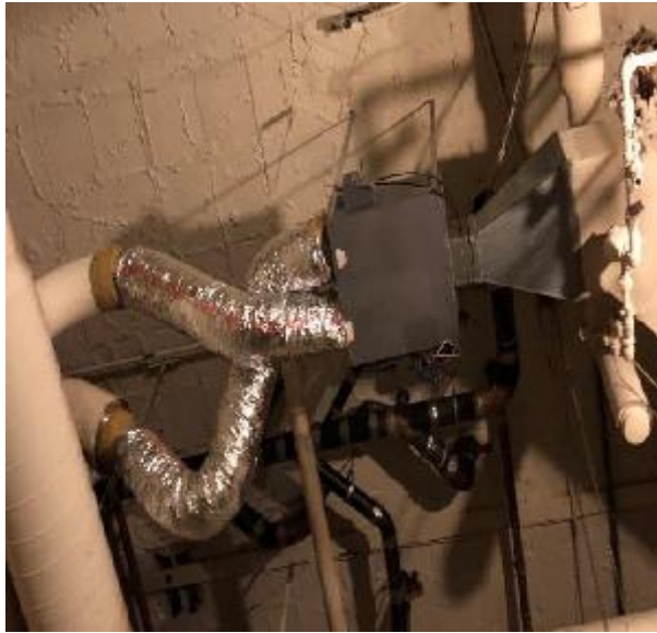
Figure 15: Original dual duct box
