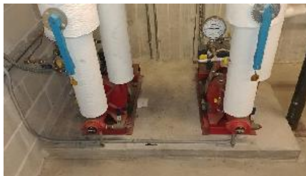
Figure 28: Existing Hot Water Pumps
