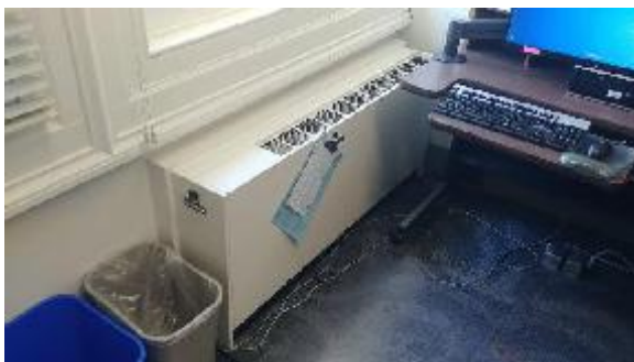
Figure 21: Existing Fan Coil unit (Exterior)
