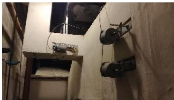
Figure 10: AC-7 zone control dampers
