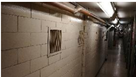
Figure 11: AC-7 supply grilles in space
