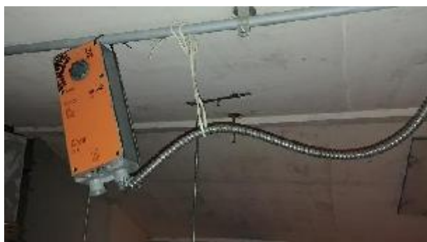
Figure 36: AHU-2 Actuator, disconnected.
