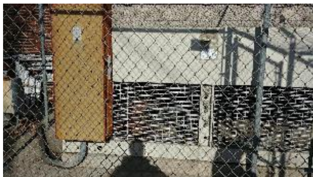
Figure 37: ACCU-1 outdoor unit, with rust.
