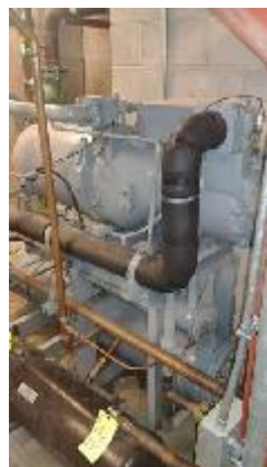
Figure 41: Existing DX screw compressor unit.
