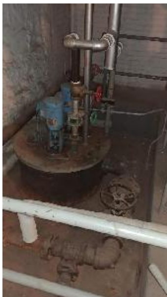
Figure 26: Existing condensate receiver for the building.
