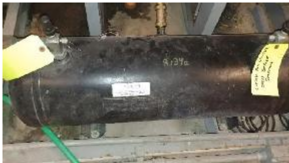
Figure 39: DX system Evaporator bundle
