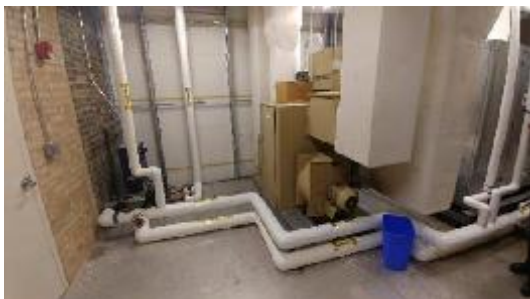
Figure 25: Rare books Desiccant Dehumidification system.
