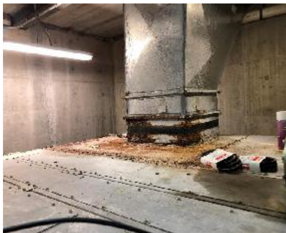
Figure 30: AHU-1 OA duct with significant rust.
