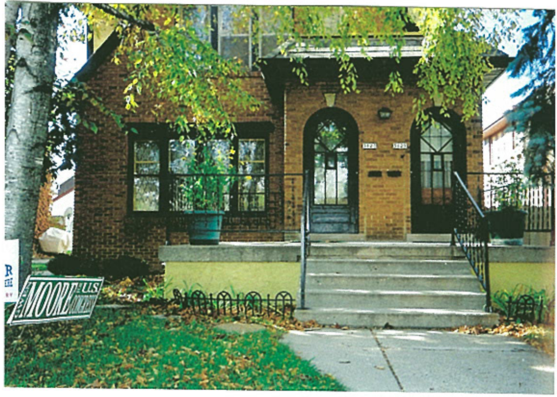
2. ORIGINAL STORM DOORS, WINDOWS AND SCREEN DETAIL
