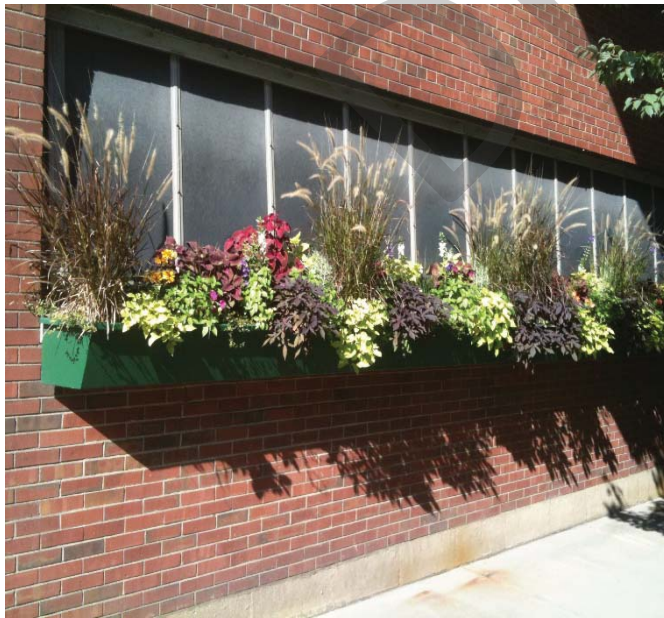
Facade, landscape, and streetscape improvements at A. Finkl & Sons Company steel forge. Clockwise from upper left: Street and accent lighting; industrial archways found at the industrial park gateways; window boxes with ornamental plantings.
