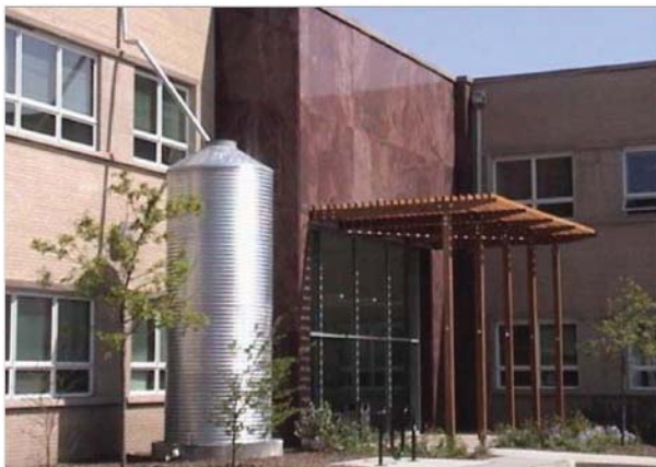
Lowest ranked stormwater image.
