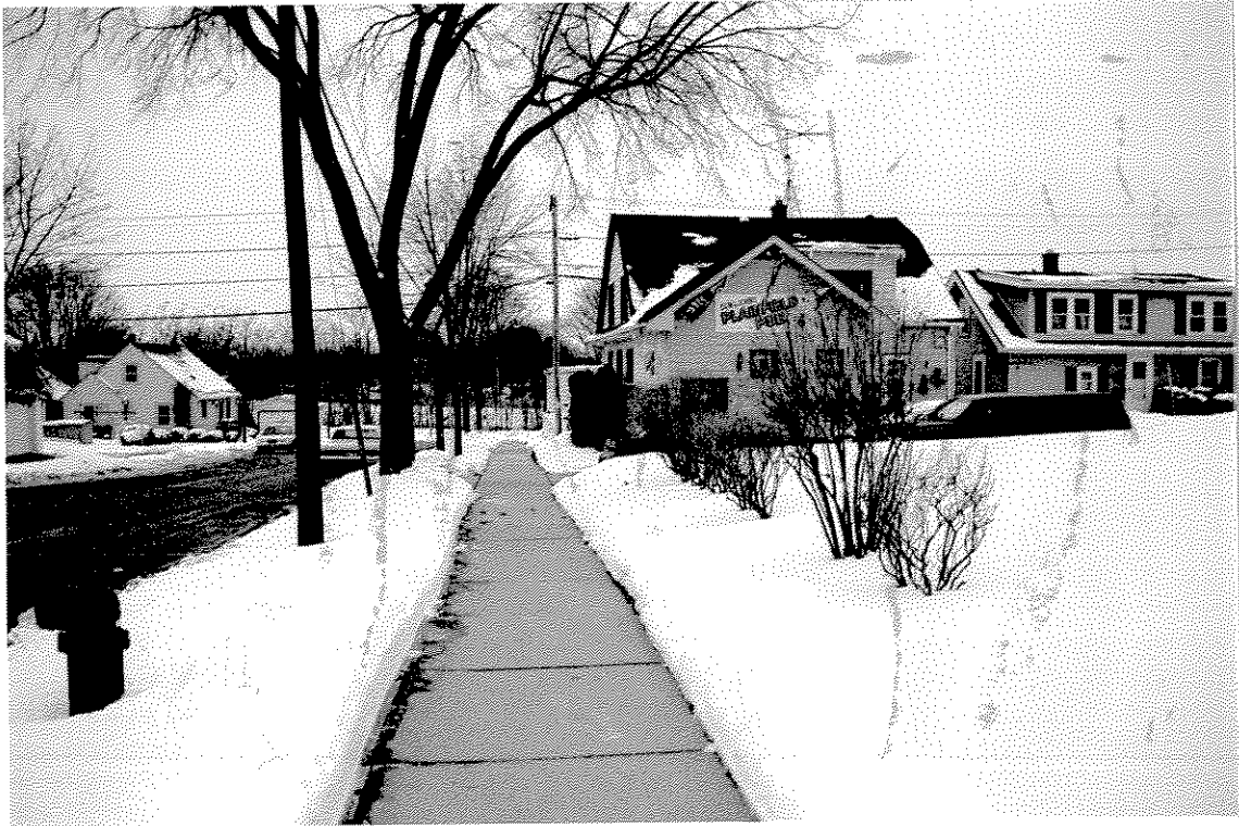
View #1 NW Corner of 3 rd and Plainfield, facing west
