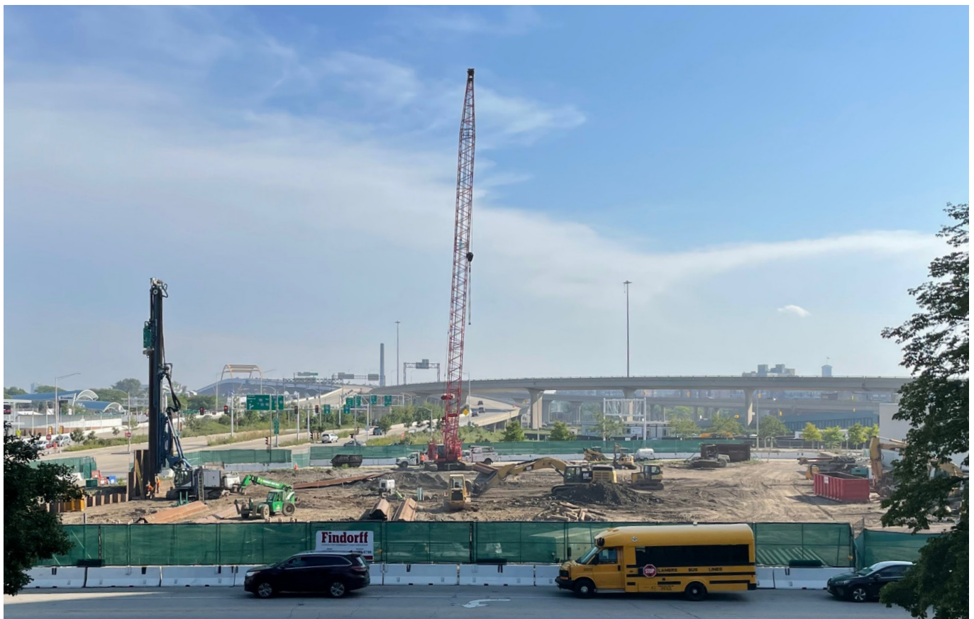
Sewer work site.
