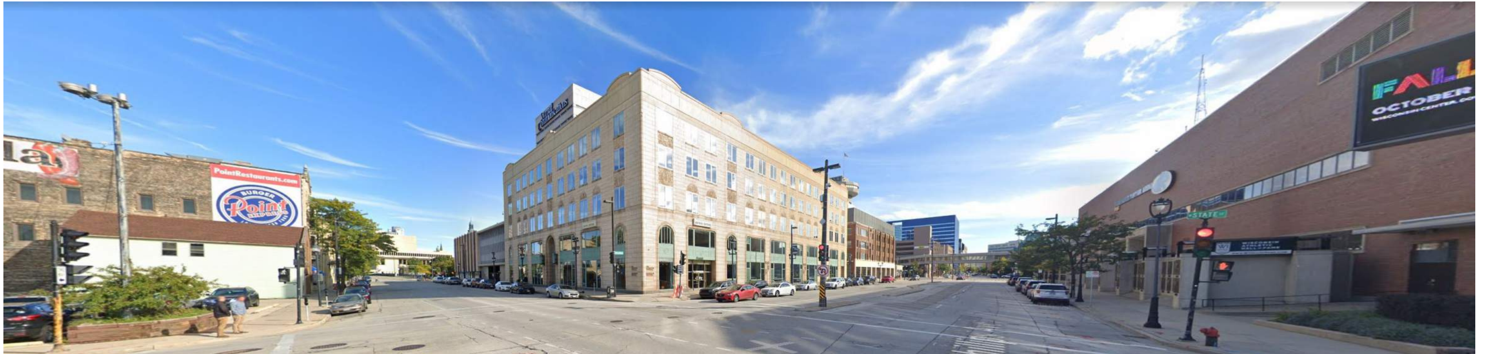
N. VEL R. PHILLIPS & STATE STREET LOOKING SOUTHEAST
