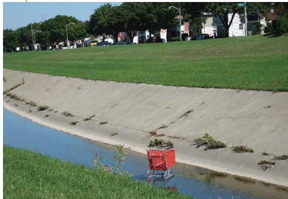
KK concrete channel
