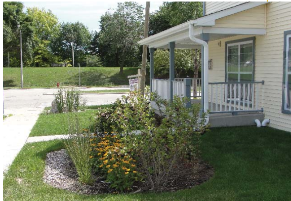
HACM home with rain garden
