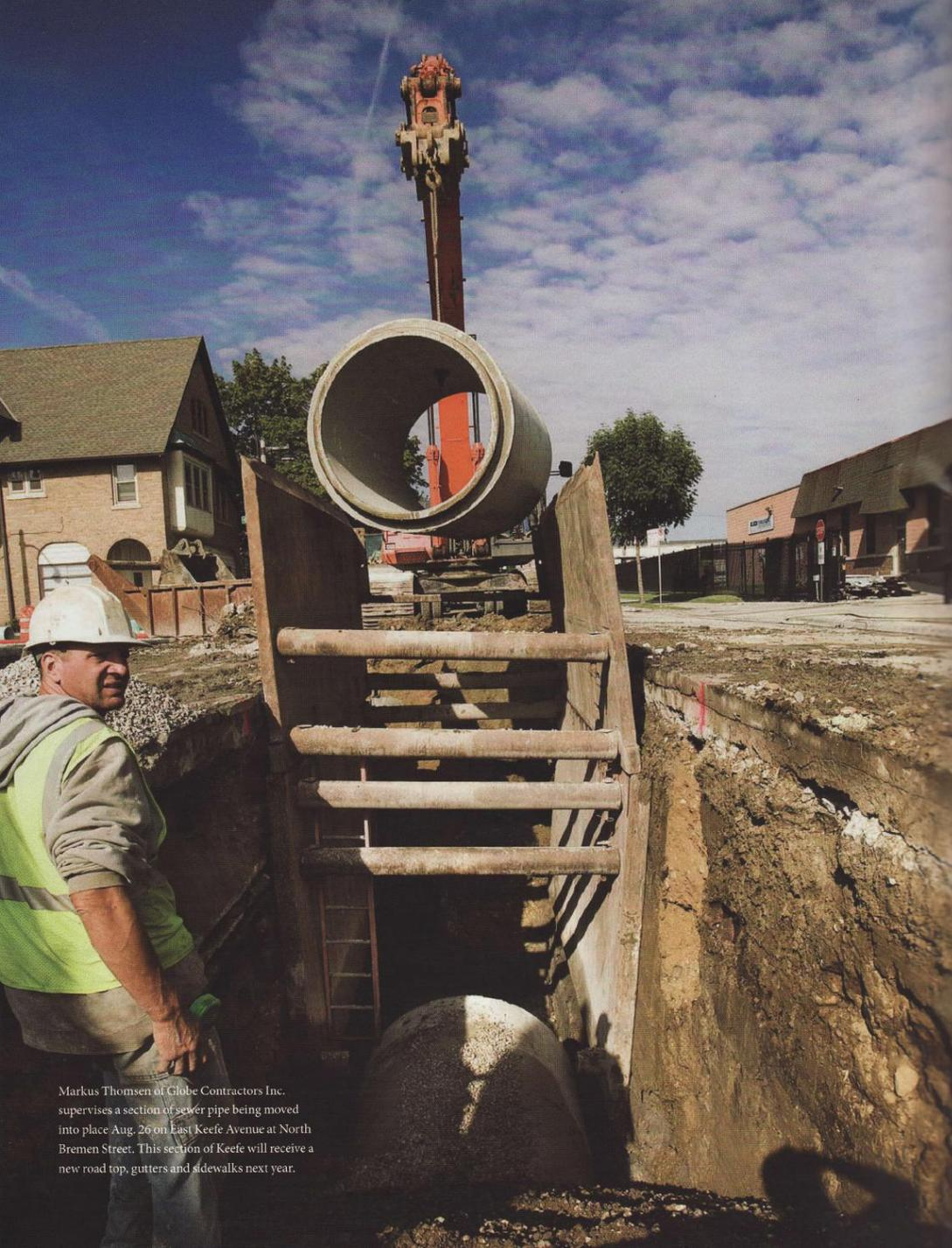
Markus Thomsen of Globe Contractors Inc. supervises a section of sewer pipe being moved into place Aug. 26 on East Keefe Avenue at North Bremen Street. This section of Keefe will receive a new road top, gutters and sidewalks next year.
