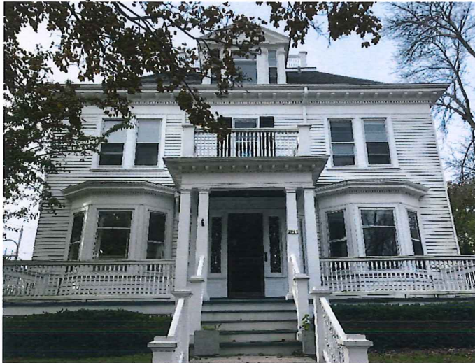
North Façade – 2803 E Bradford Ave
