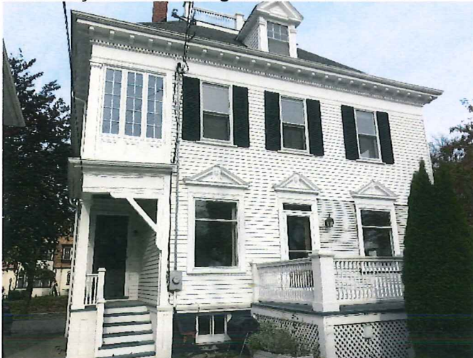
East Façade with Fiberglass Door & Transom
