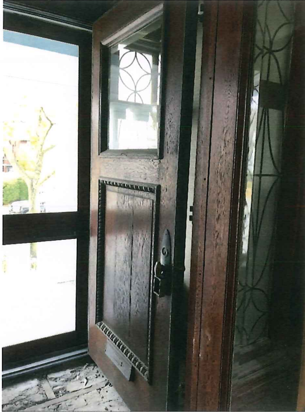
Existing Front Door
