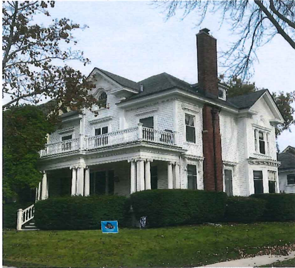
2734 E Bradford, South & East Facades
