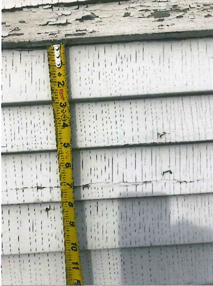
Existing Photo of Original Siding under Vinyl Siding
