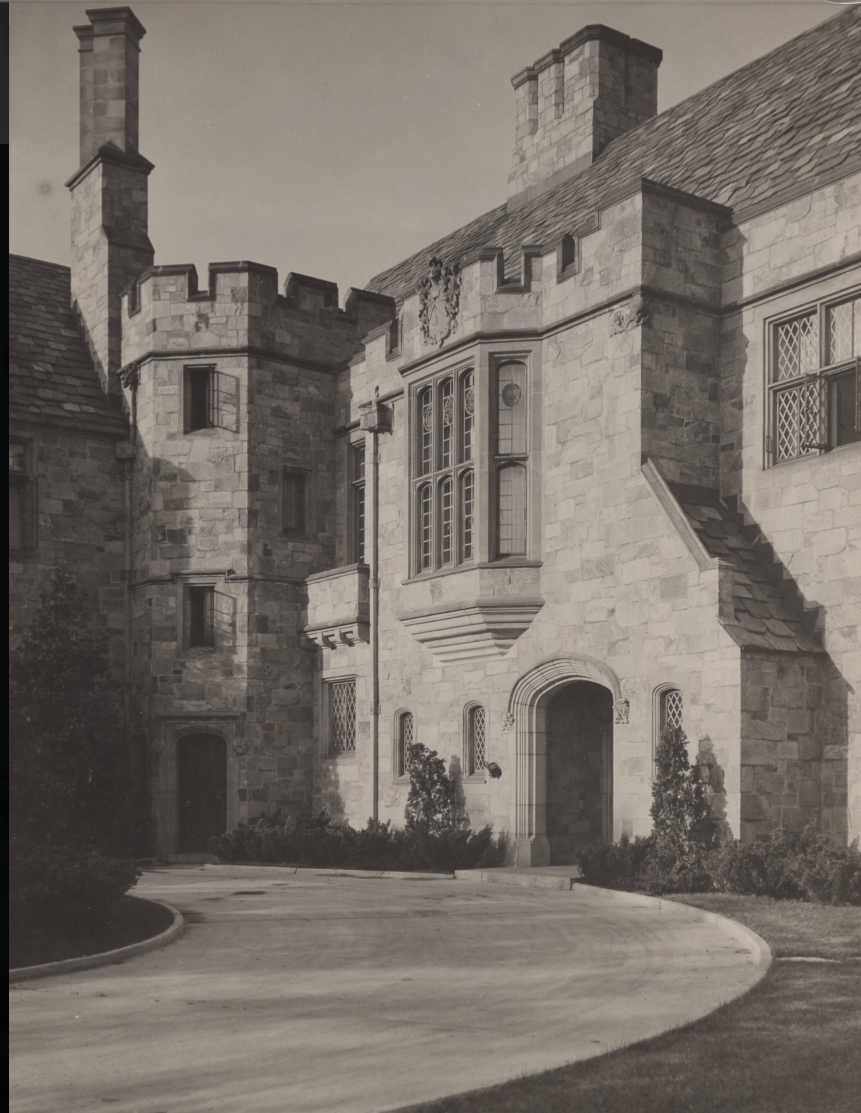
1925 Photo of Myron T. McLaren House (original placement of concrete circular drive)
