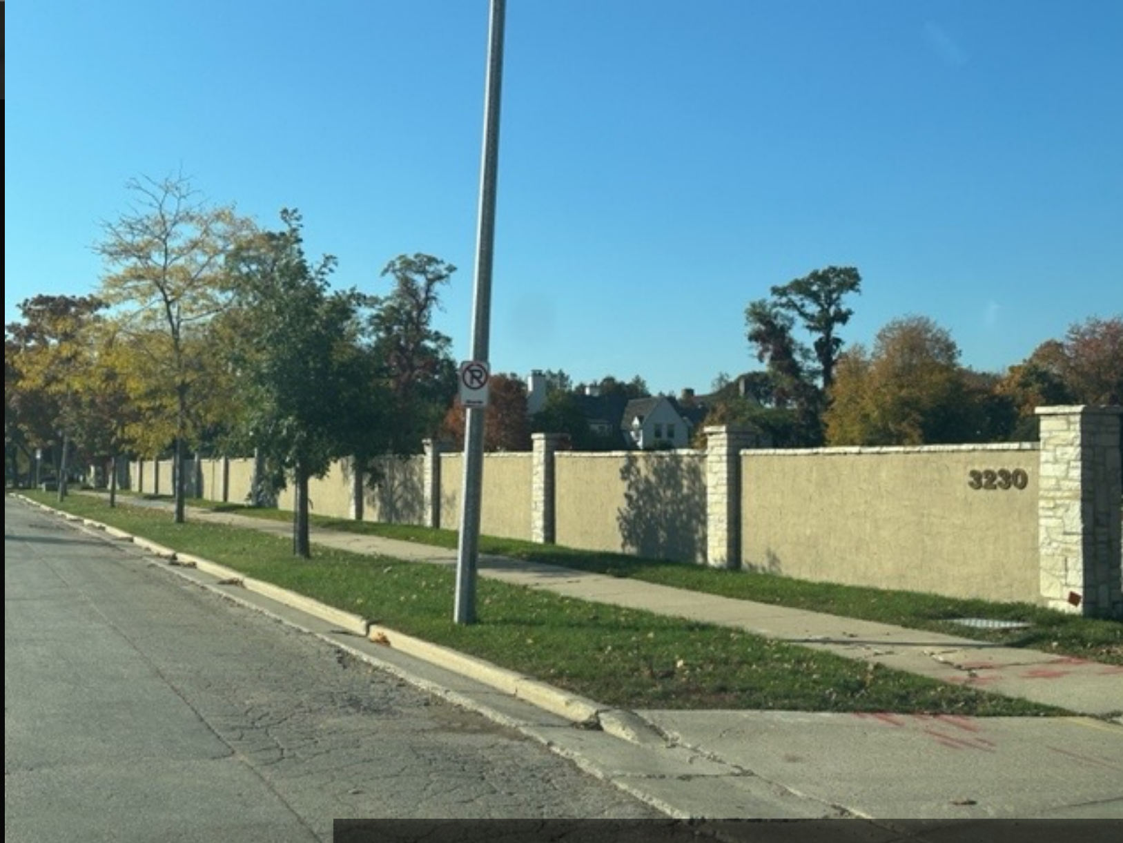
Northwest street view (Kenwood Blvd) of current wall.
