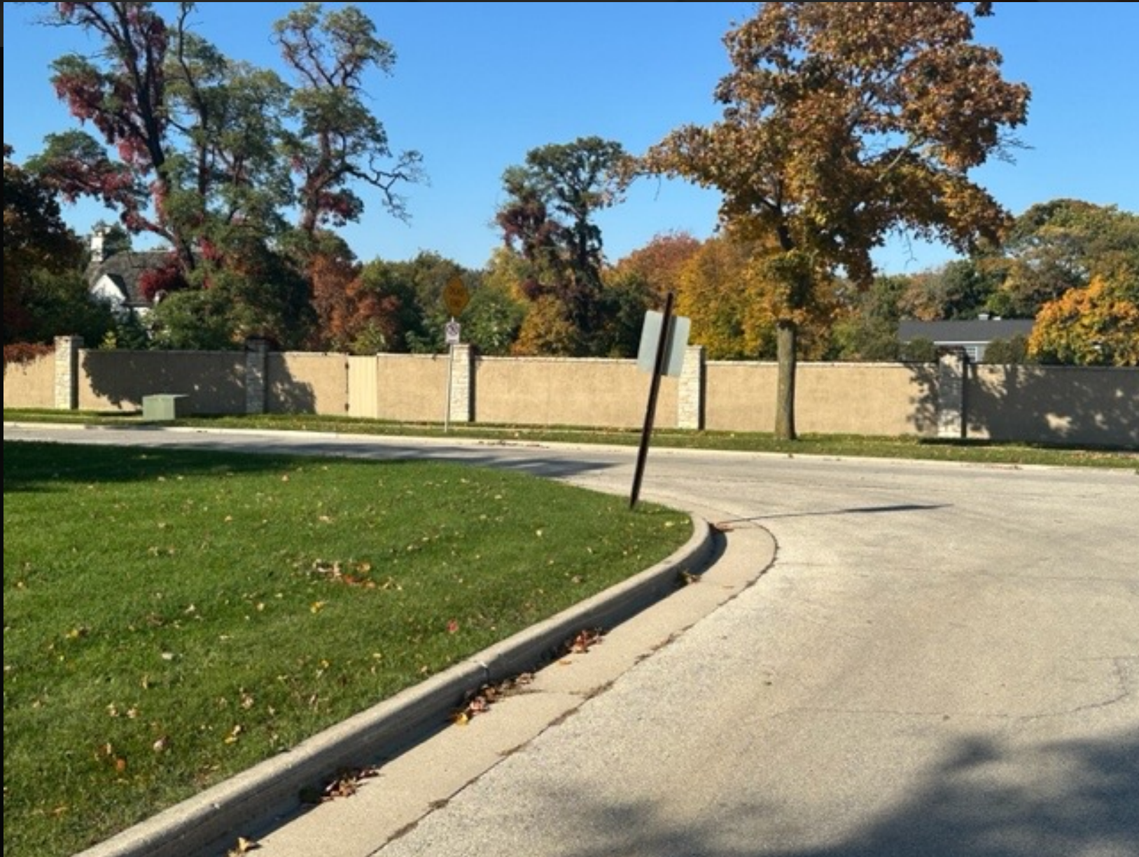
View northward from Lake Park Drive of current wall
