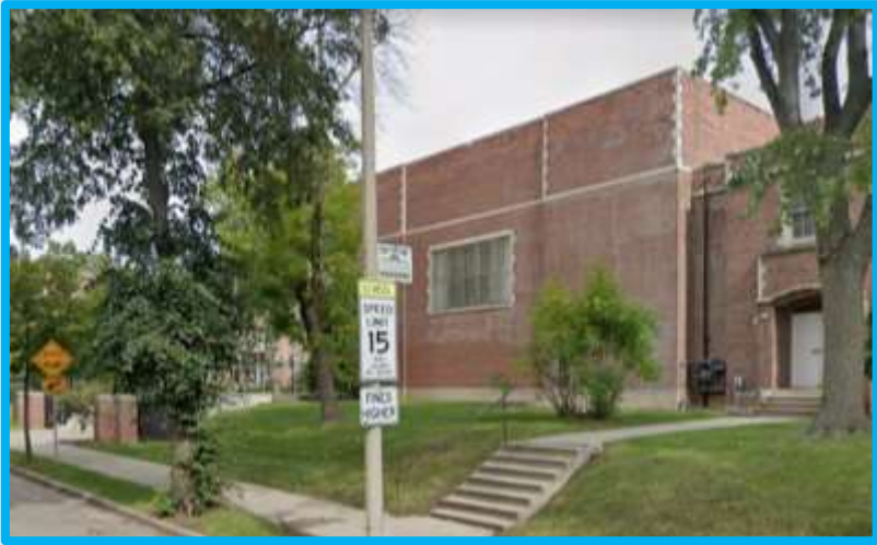
View from N. 33 rd St. looking northeast
