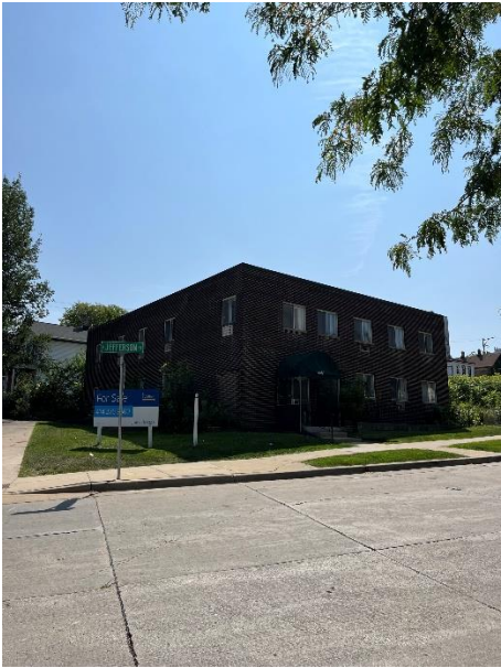
Existing office structure onsite. View looking east.
