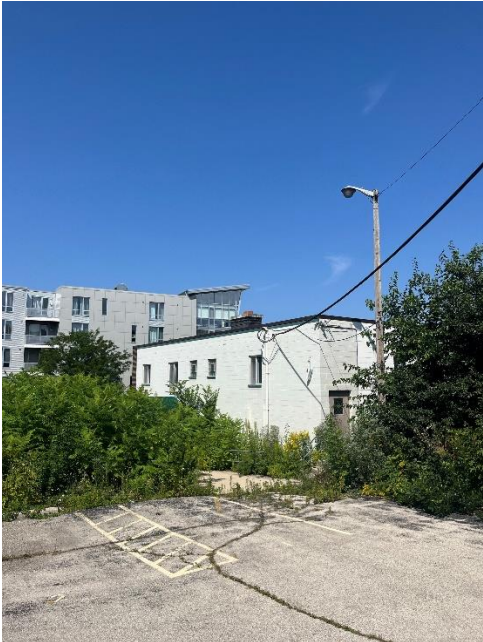
Existing office structure onsite. View looking northwest.
