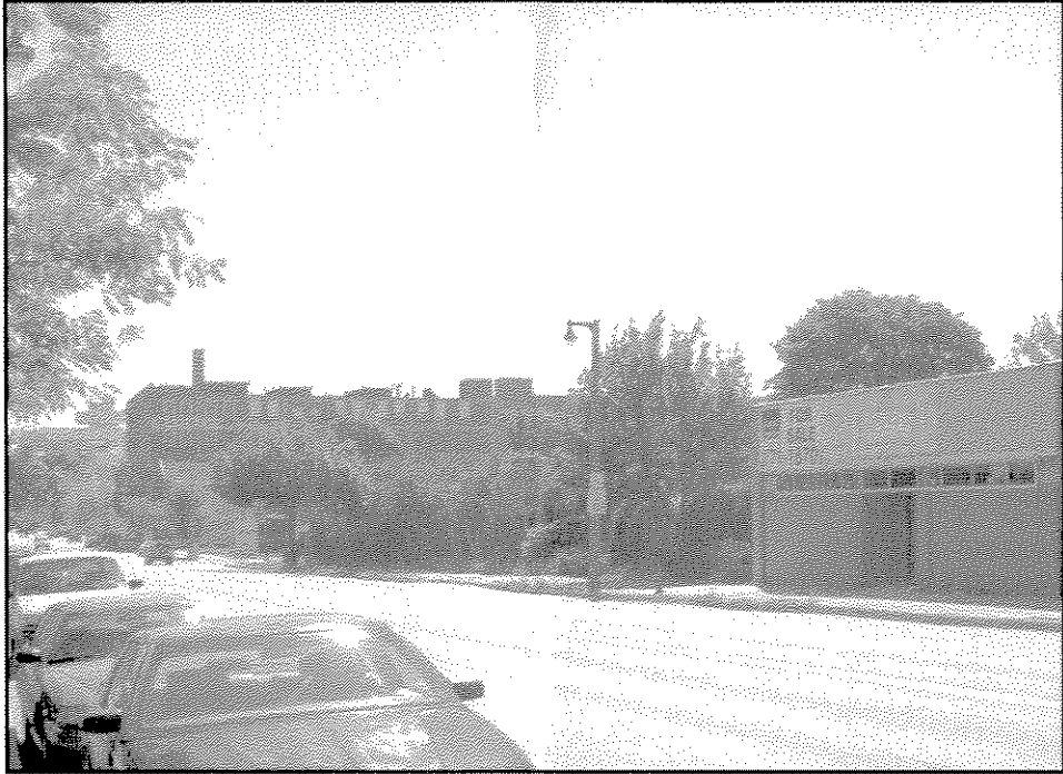
Looking southwest from Martin Luther King Jr. Dr. across site. Shows vacant building (right side of photo) that will be demolished as part of development.
