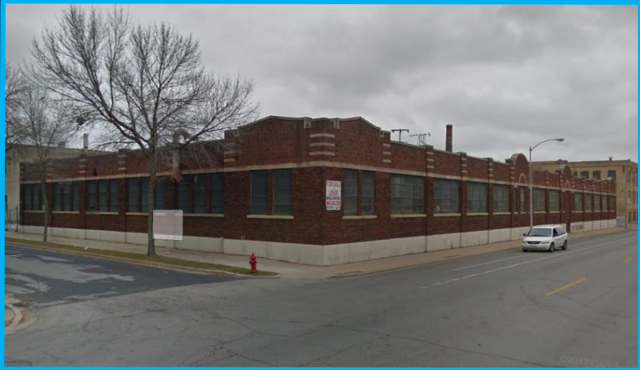
View from West Center Street and North 33 rd Street
