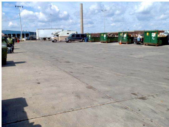
Self Help concrete
