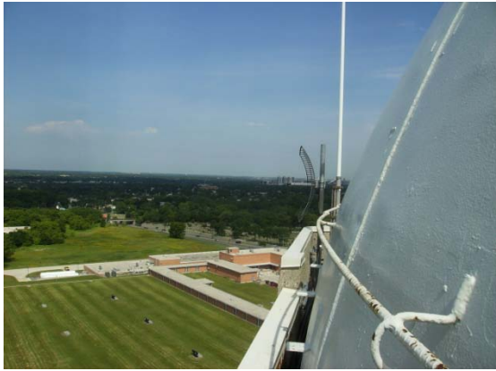
Parapet wall, antenna, and water tank
