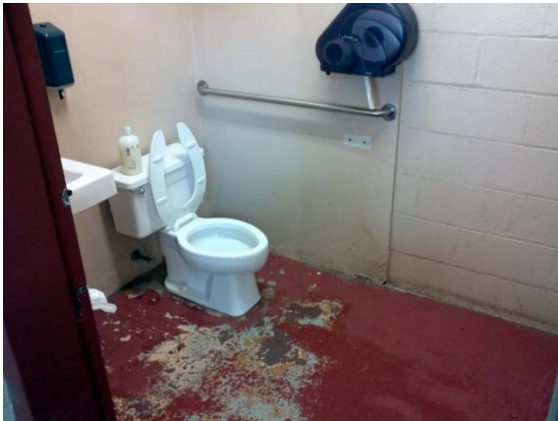
Stand alone rest room finishes
