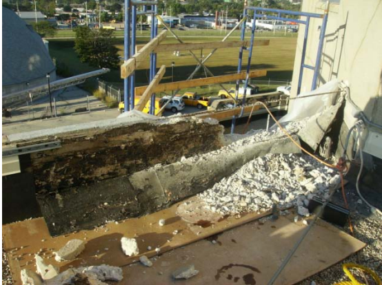
3 rd floor parapet wall rebuild
