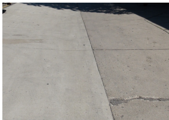
Partial concrete replacement
