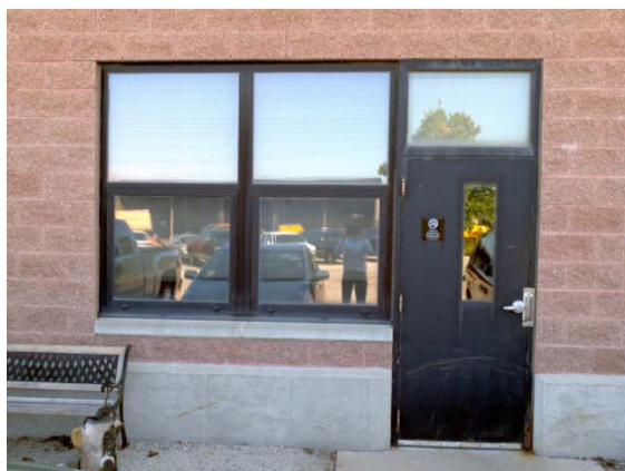
Typical frame window installation
