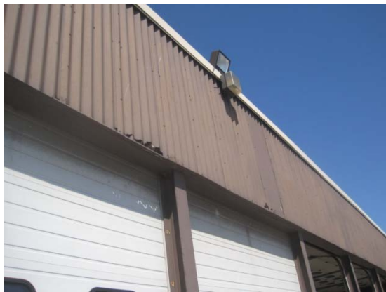
Garage light fixtures
