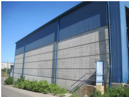
Gutters and downspouts
