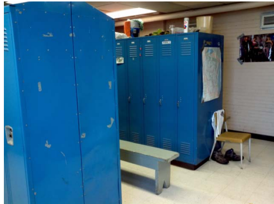
Men's rest room finishes
