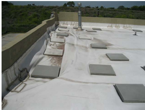
Roof 6 adhered with pavers
