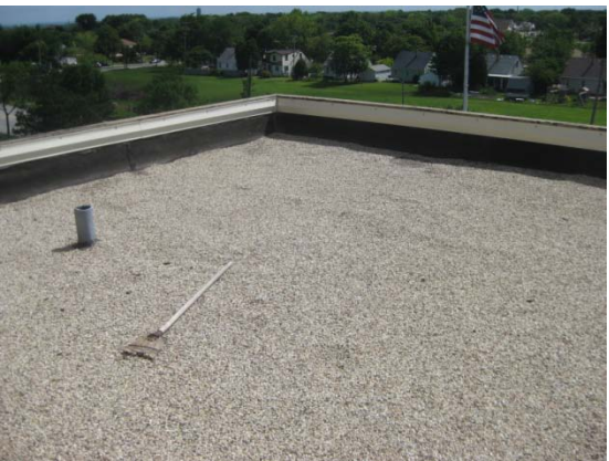
Roof 1 w gravel ballast
