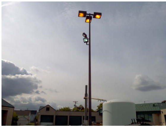
Light pole and fixture
