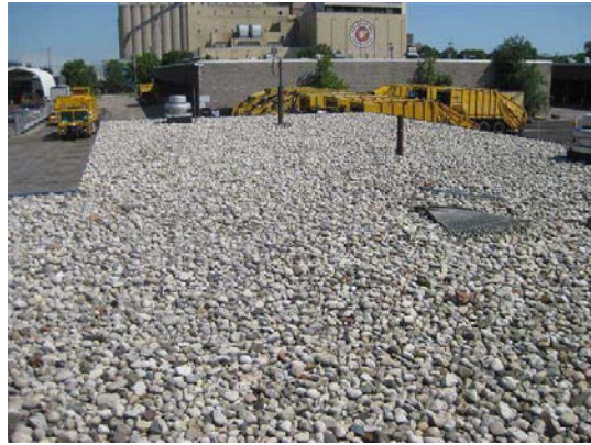
Scale House roof
