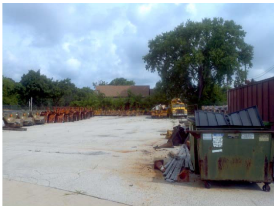
Typical asphalt pavement
