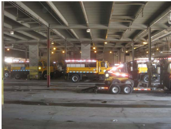
Steel components – Lincoln Garage
