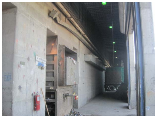
Typical Lincoln Garage light fixture
