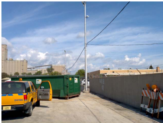
Light pole and fixture
