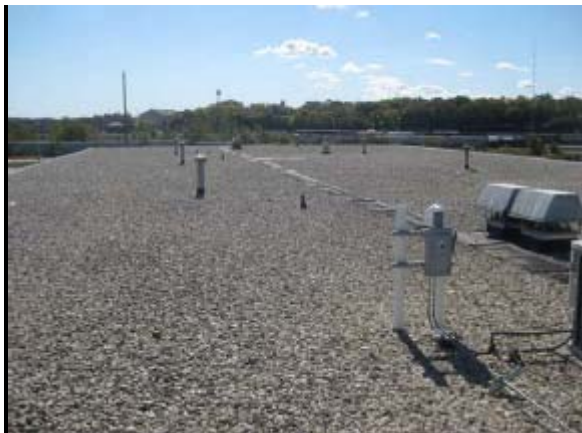
Ballasted EPDM roof
