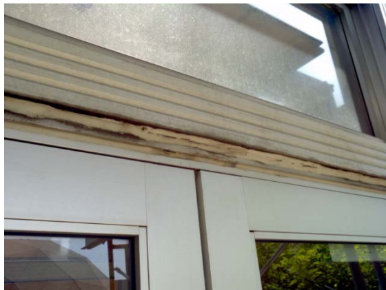
Caulk at doors replaced in 2011
