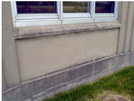
Repointed window sill
