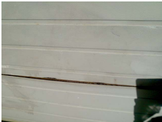
Damaged garage door panel
