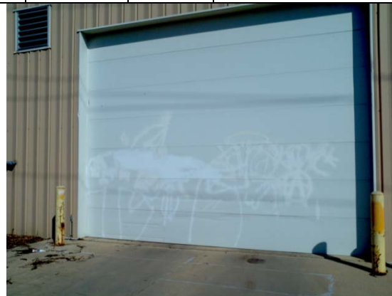
Garage door at Storage Garage
