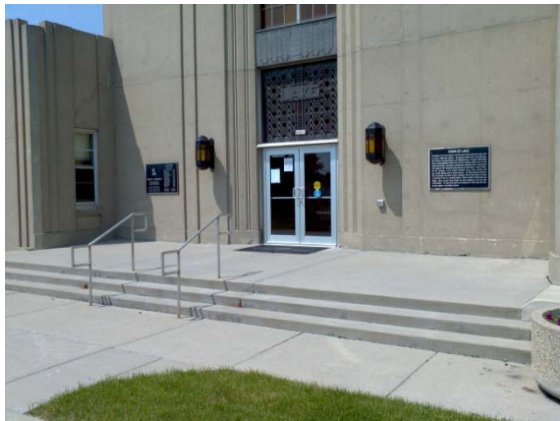
Front entrance doors
