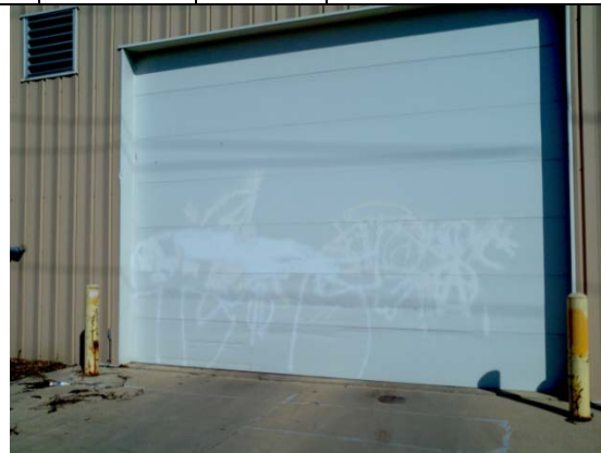
Garage door at Storage Garage
