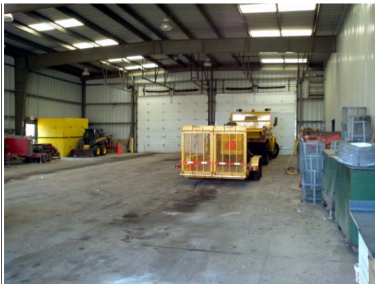
Metal roof w translucent panels
