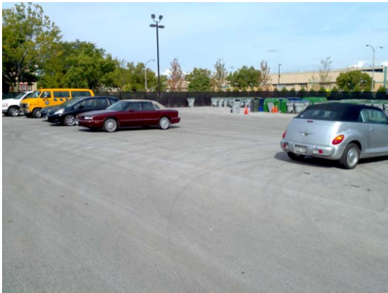
Northwest pavement – relatively good condition
