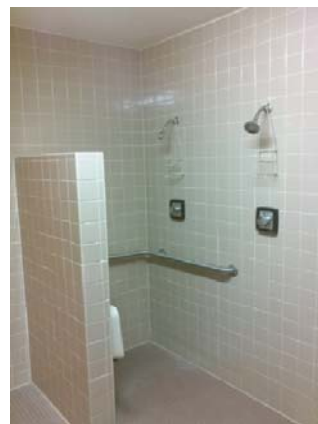
Men's shower finishes
