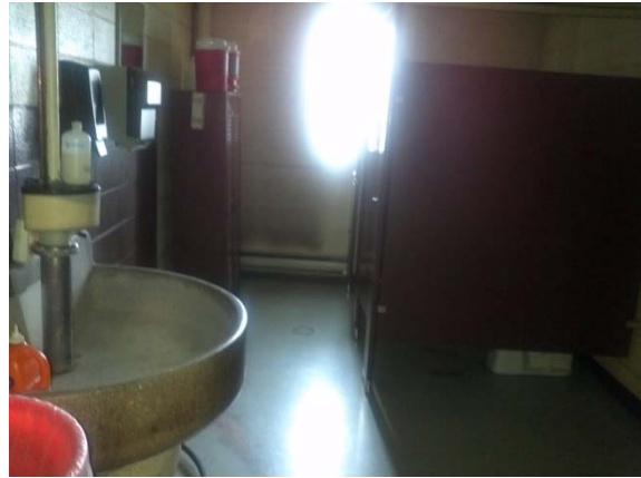
Large rest room
