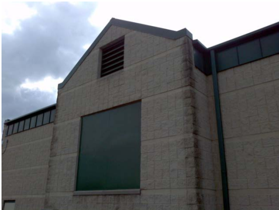
Panel siding and fascia
