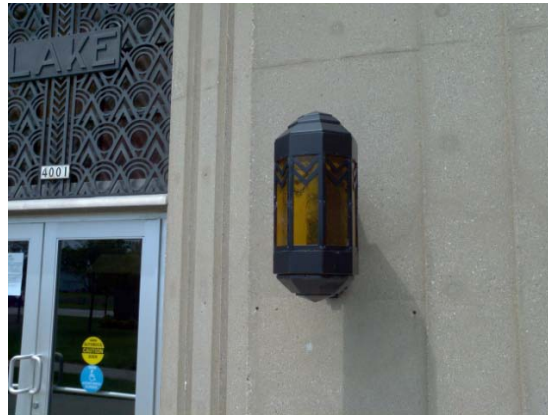
Typical light fixture
