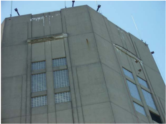
Concrete eyebrow restoration
