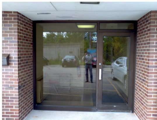
Glass entrance door
