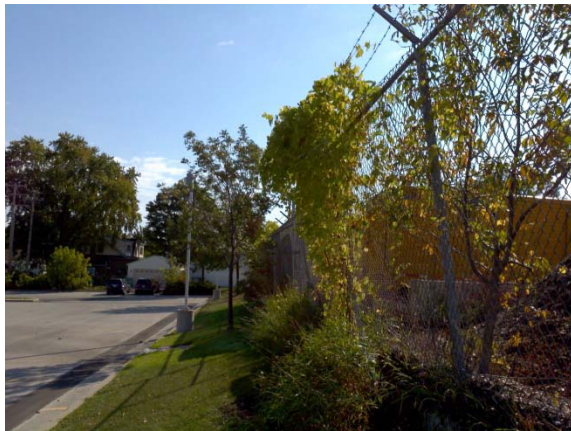
Misaligned fence at north perimeter
