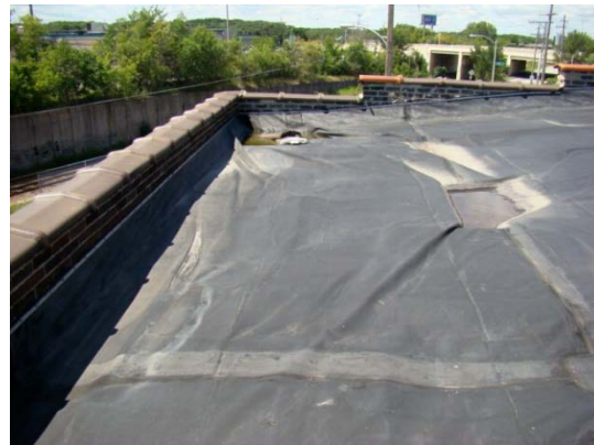
Floating insulation underneath membrane
