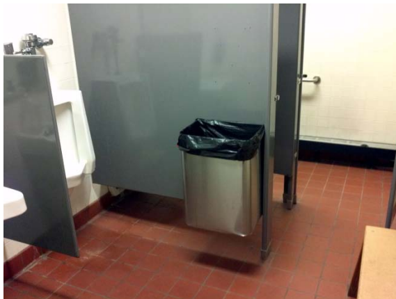
Typical rest room interior finishes
