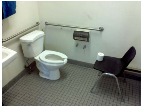
Scale house rest room finishes
