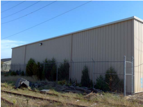
Gutters and downspouts at west elevation
