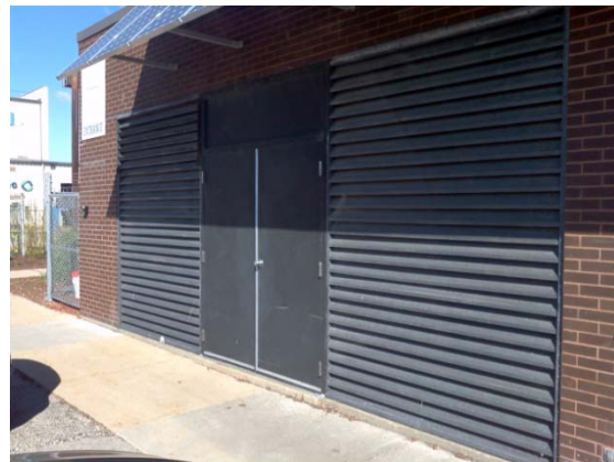
Metal doors and louvers
