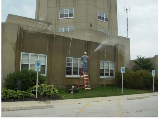
Concrete sealer application
