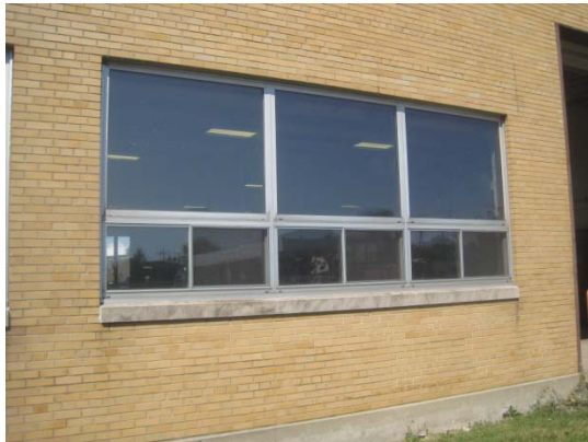
Lincoln Garage windows
