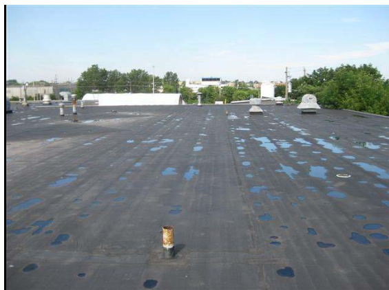
Lincoln Garage roof overview
