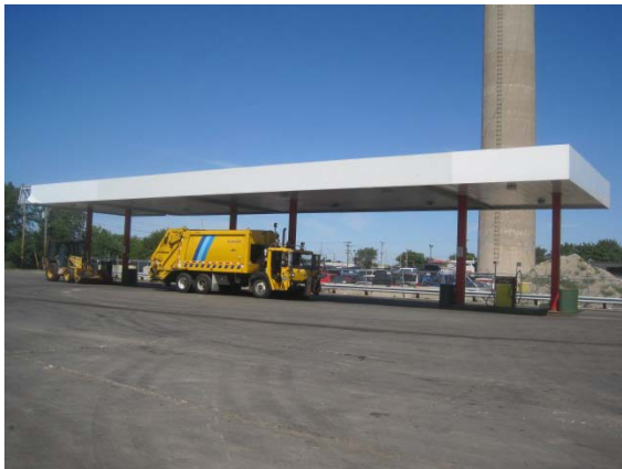
Southwest fuel island
