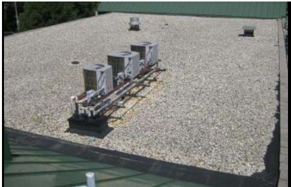
Ballasted EPDM roof
