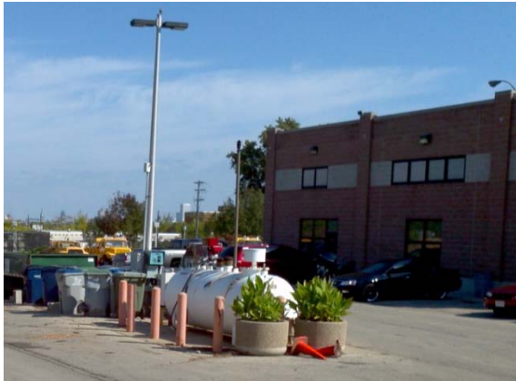
Gasoline fuel station
