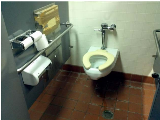
Rest room finishes
