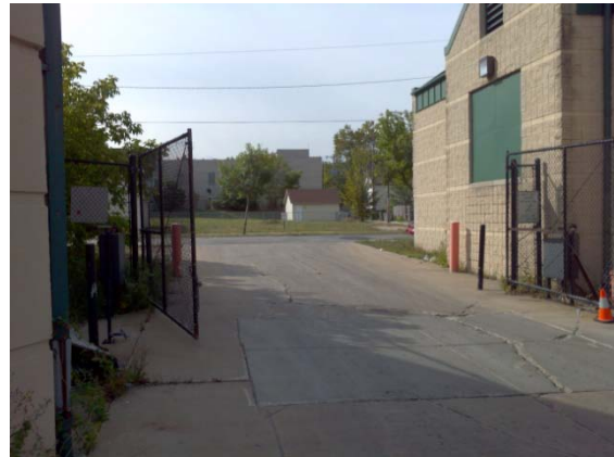
Gates and operators
