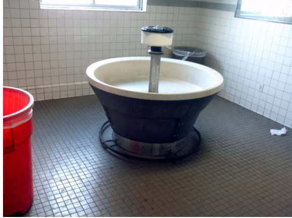
Rest room finishes
