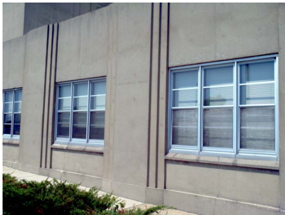
Typical aluminum frame windows
