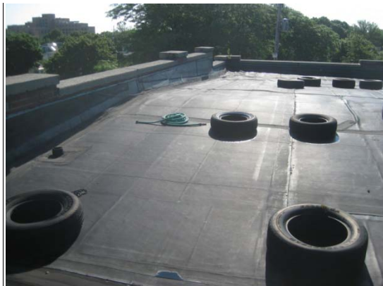
Roof #1 - tires restrain membrane
