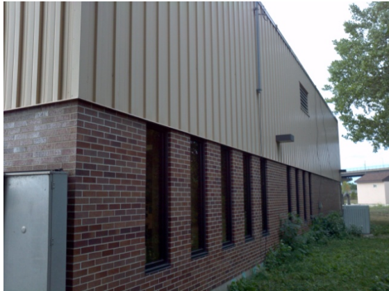
Typical aluminum frame windows at north elevation
