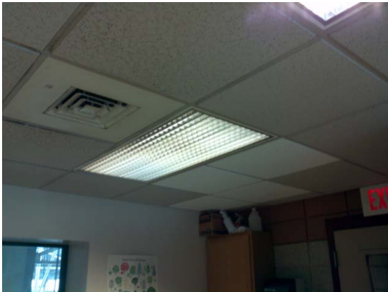
Replaced ceiling tile 2 nd Floor offices
