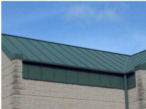
Gutters and downspout
