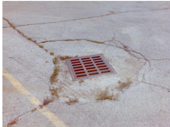
Catch basin with minor settlement
