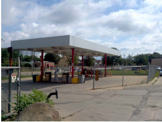
Northeast fuel island
