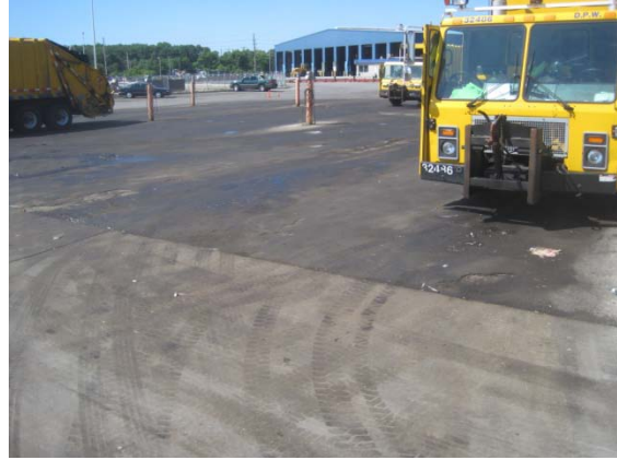
Lincoln Garage asphalt pavement
