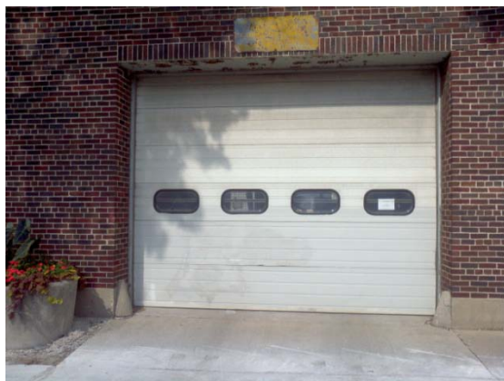
Typical garage door
