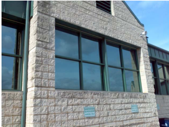
Typical aluminum frame windows
