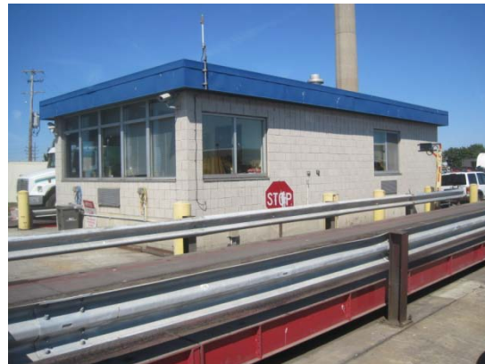
Scale House windows
