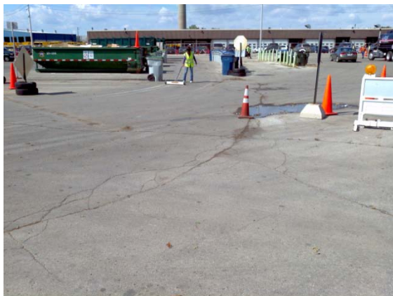
Asphalt pavement at Self Help
