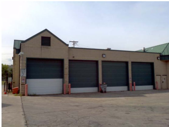
Office building garage doors
