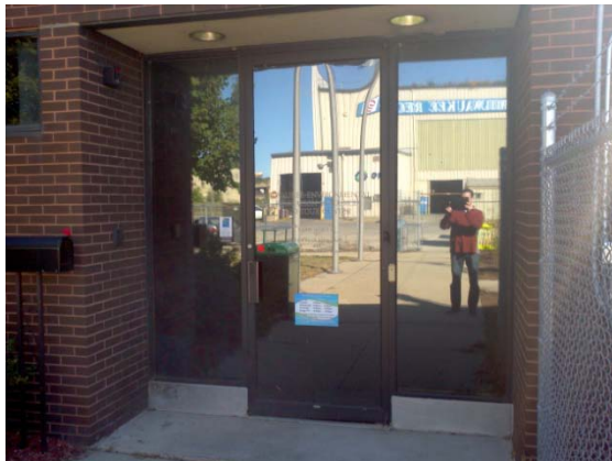
Glass/aluminum framed windows/doors
