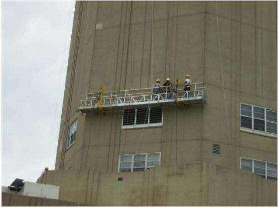
Swing stage rigging
