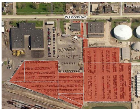
Typical cracked pavement at west lot
