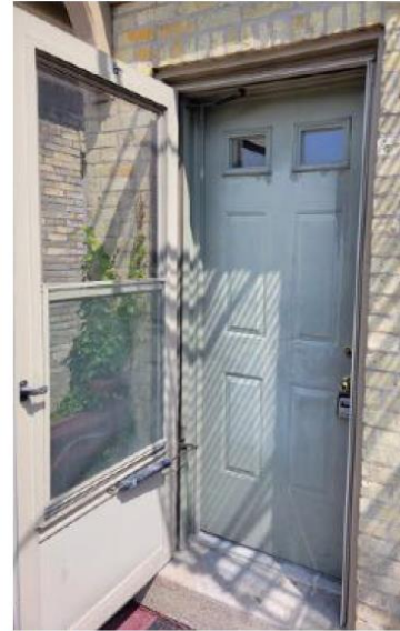
IMAGE 10: Current second floor west (rear) door.
