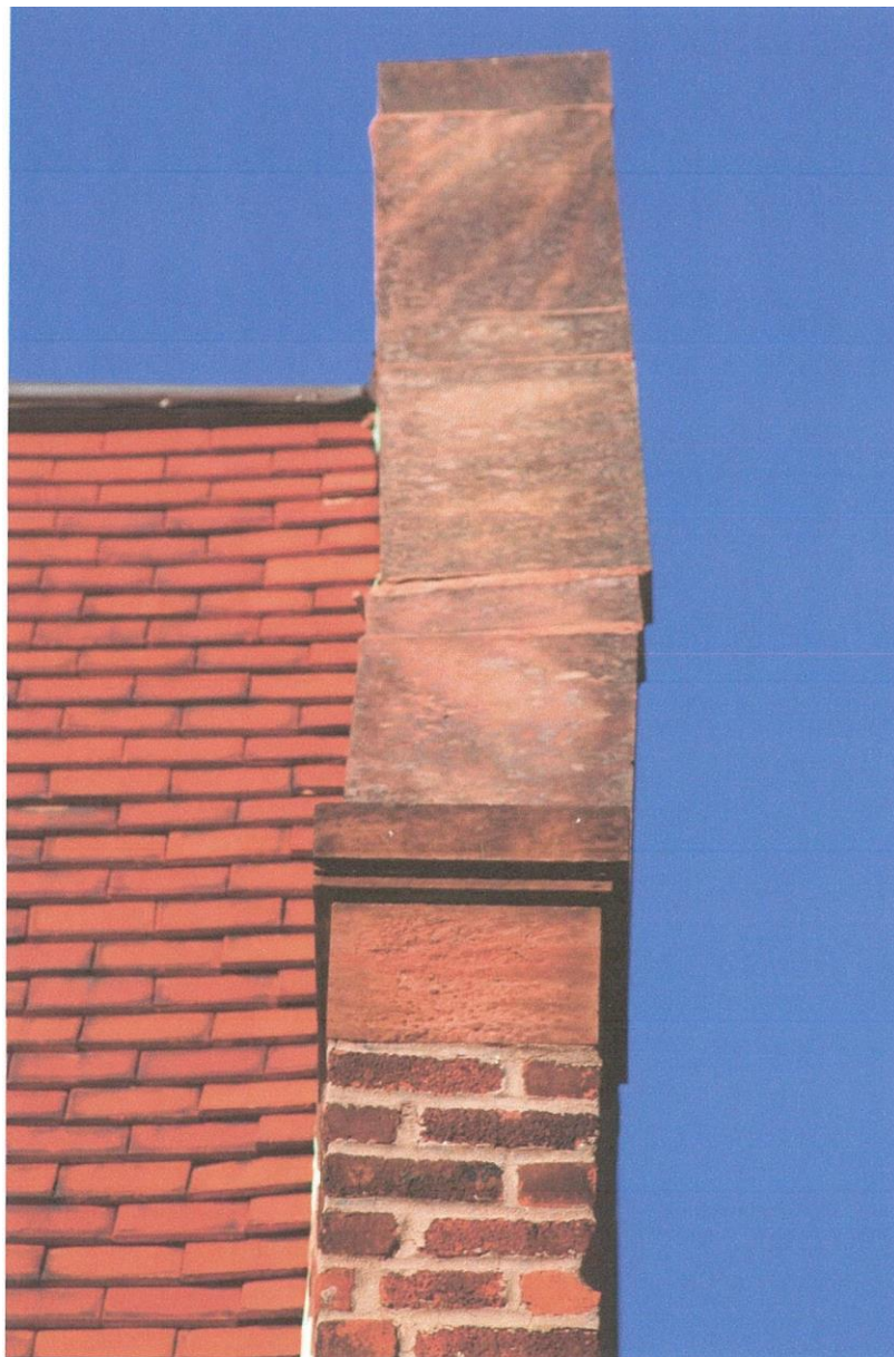
Leaning parapet and displaced gable coping – NE corner – Charles Allis House. Condition is typical to all of the gables, but to varying degrees.
