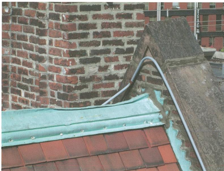
Crushed & Loose Ridge Cap – NW corner of Charles Allis House. Note excessive use of sealant on flashing, brick, and coping.
