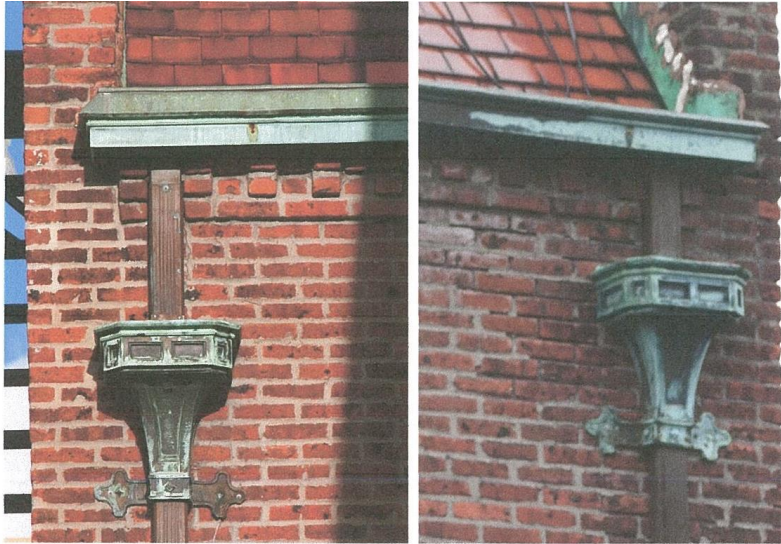
Existing Gutters – SE & NW Corners of Charles Allis House. It is proposed to raise the outer lip of the remaining unrepaired gutters to reduce the occurrence of rain runoff overflows which are contributing to the deterioration of the masonry immediately blow and further downstream of the gutters. The previous gutter work was accomplished in the 1990s as part of the previous restoration work.
