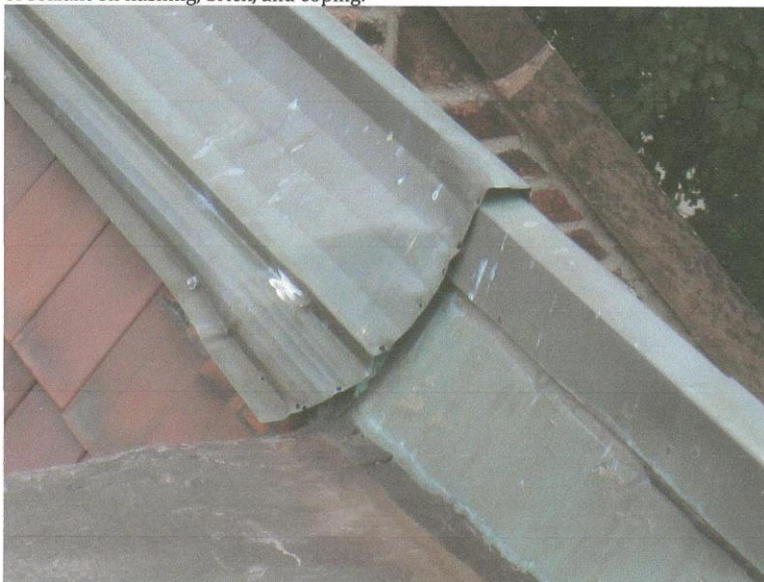
Loose Ridge Cap – NE Corner of Charles Allis House. A previous replacement, this cap was subsequently peeled open by wind or roof tile repair.
