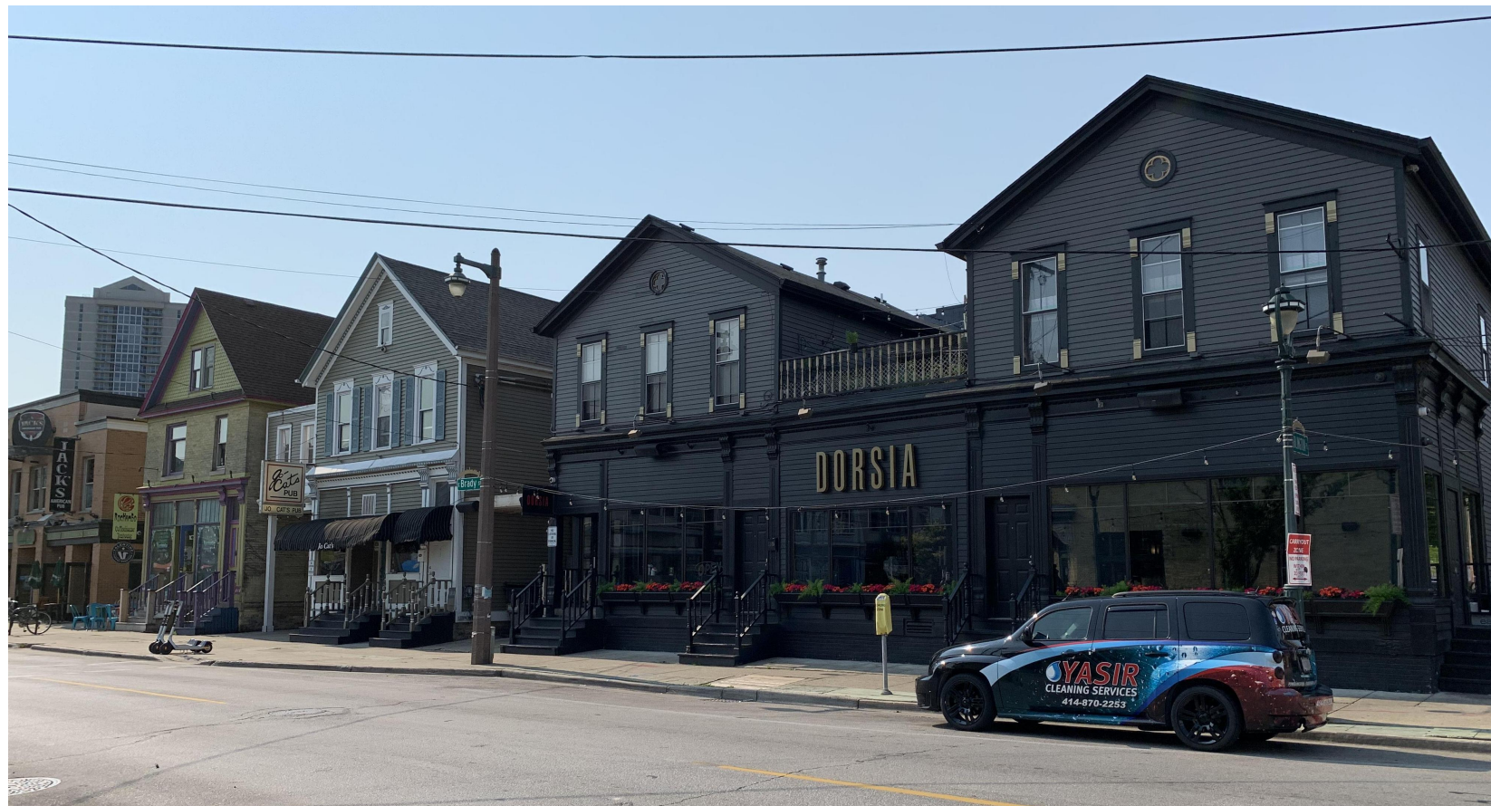
Existing Building Condition at Brady Street
