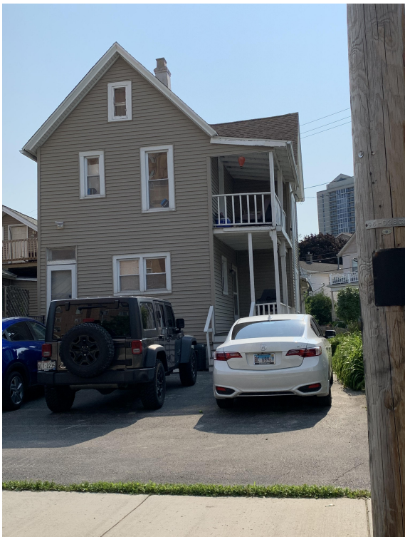
Existing Similar Building Condition - Arlington Place
