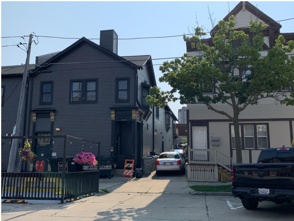
Existing Alley Condition - Arlington Place
