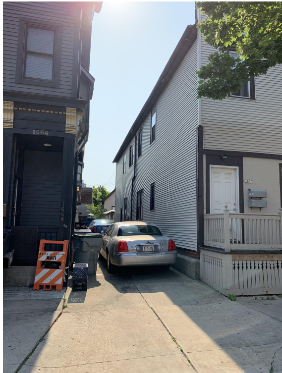
Existing Adjacent Building Condition - Arlington Place
