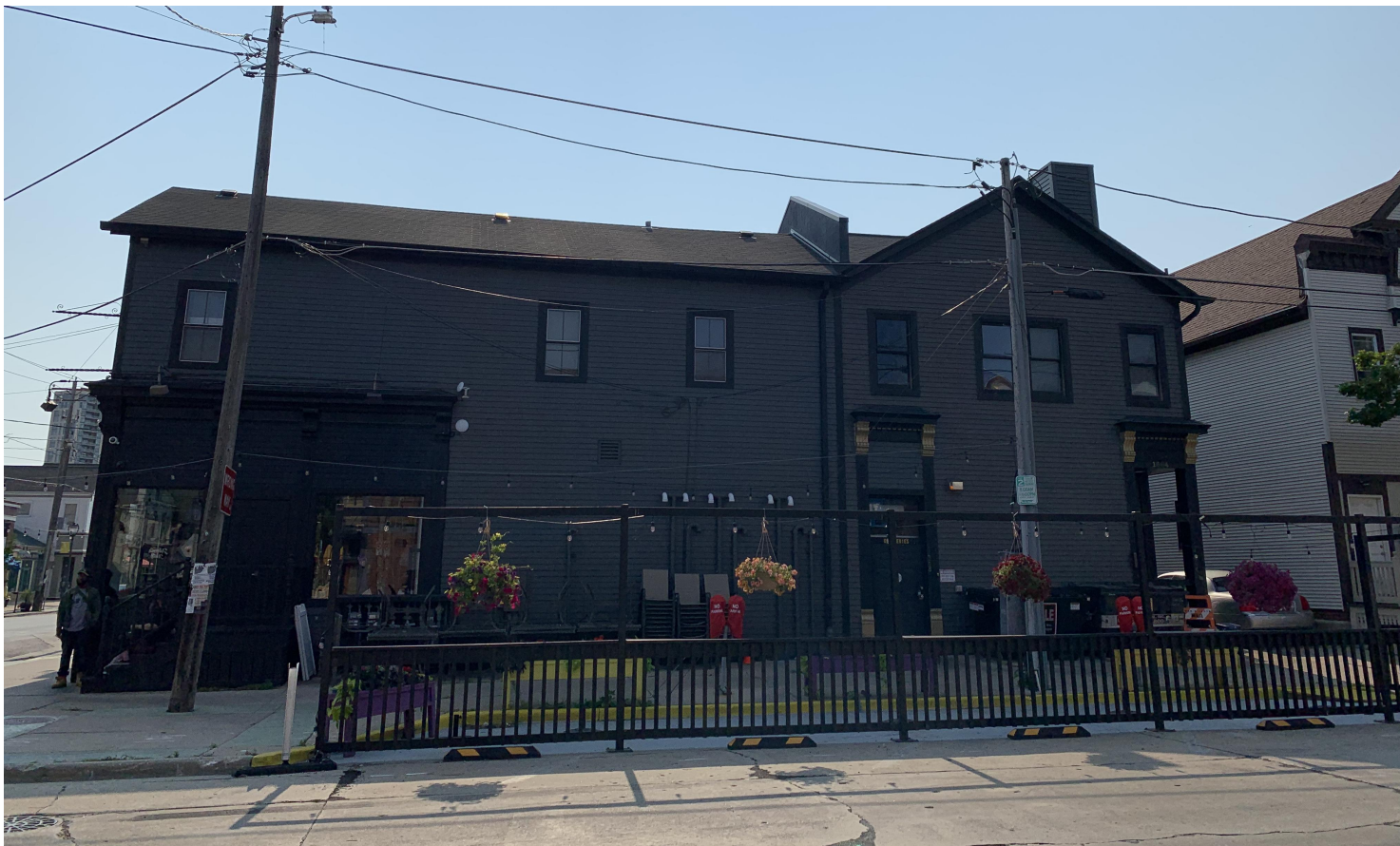
Existing Building Condition at Arlington Place
