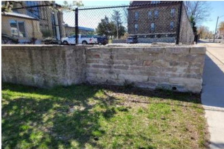
Existing stone wall at NW corner of S. 7 th Street and W. Lincoln Ave. abutting existing concrete retaining wall to the east to be clad in stone, approximately, 89LF east along W. Lincoln Avenue.
