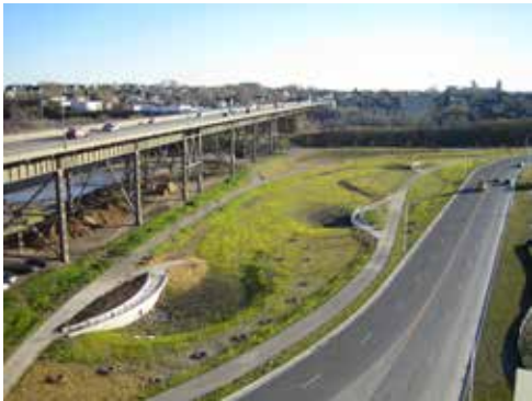
Development of Stormwater Park in MVIC manages stormwater for multiple parcels.
