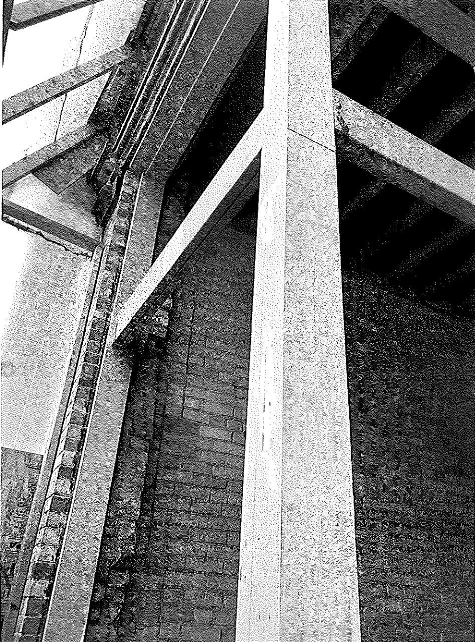
Exterior facade Southeast
