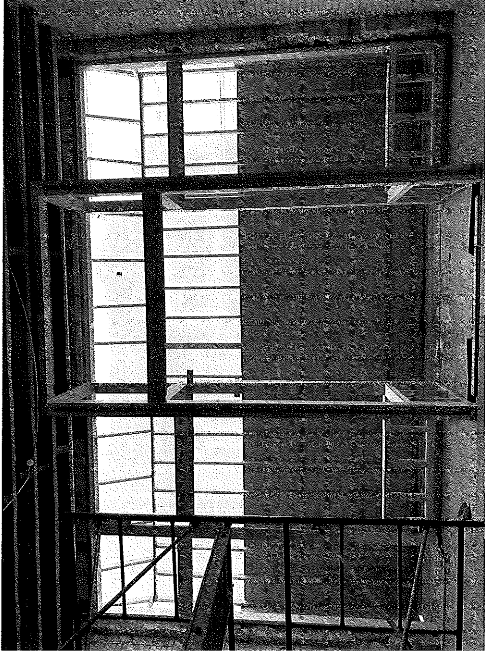
Interior Facing East
