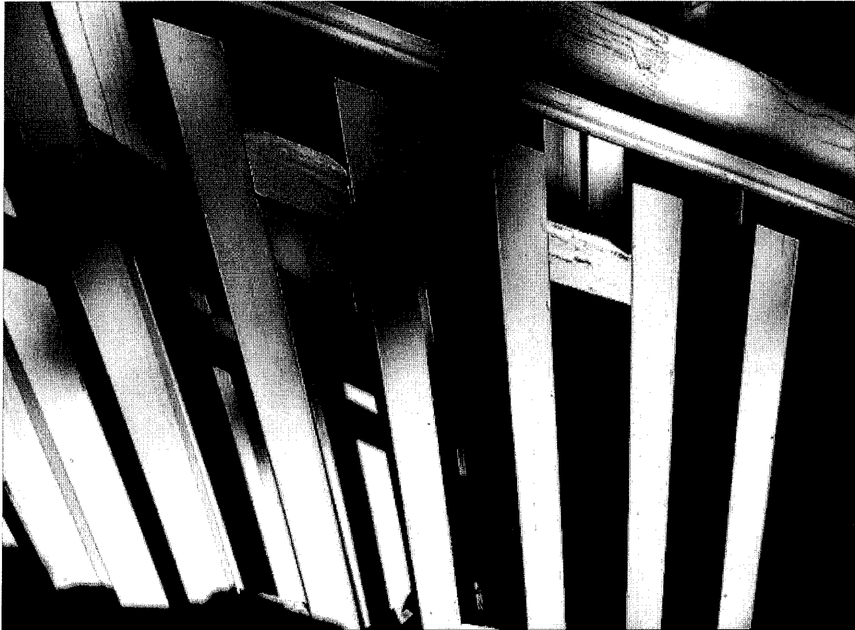
Detail of "ladder style" balustrade which will be duplicated where it presently exists and will be removed.
