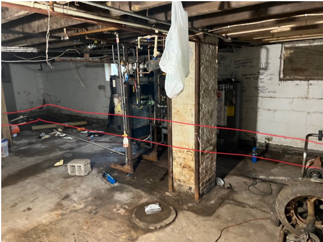
Install 100' lineal feet of 4" drain tile along the basement walls
