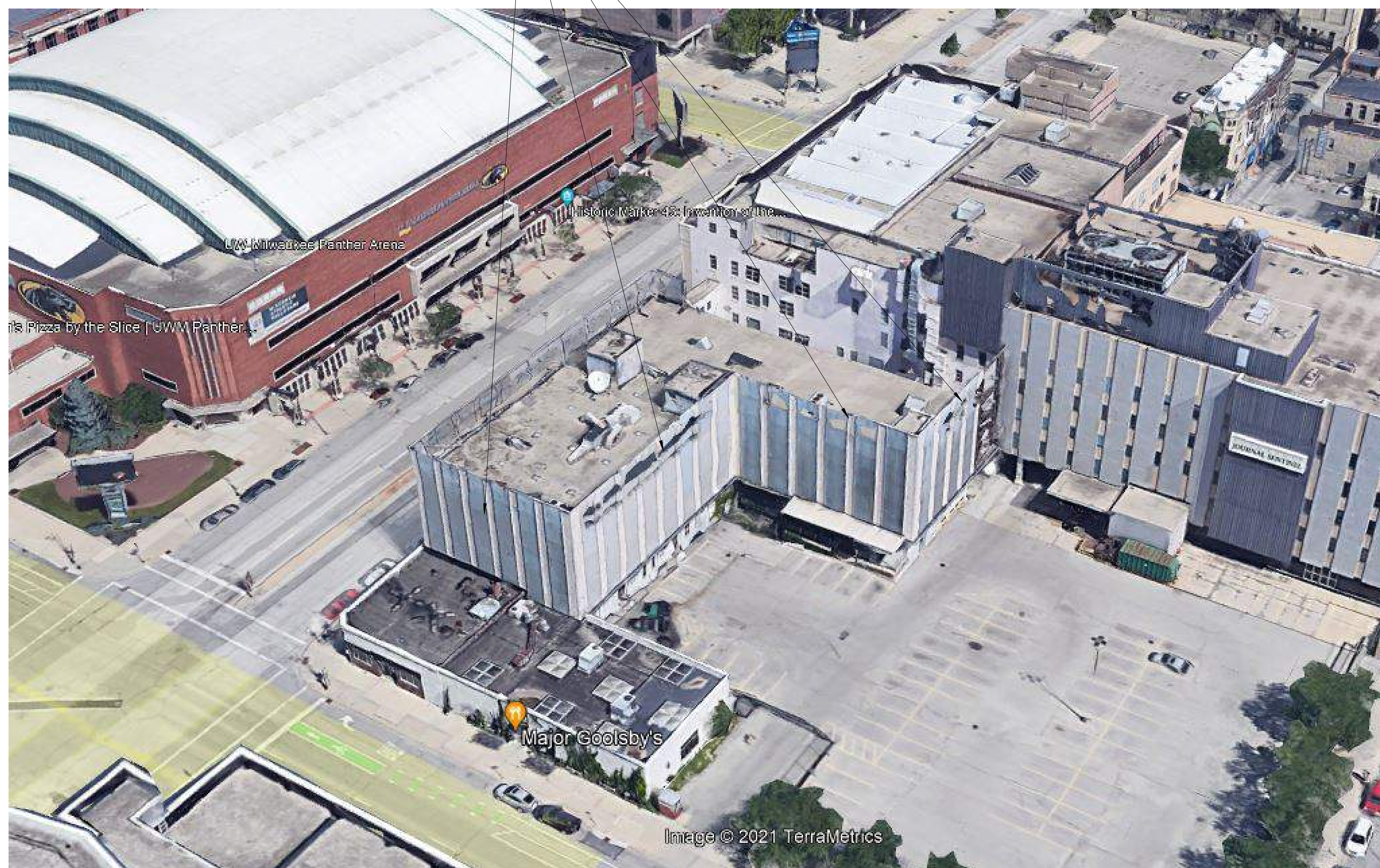
CURRENT SOUTH AERIAL
