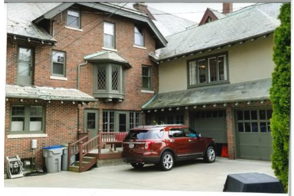
Back porch is at center left of above photo. No railing will be constructed at this time.
