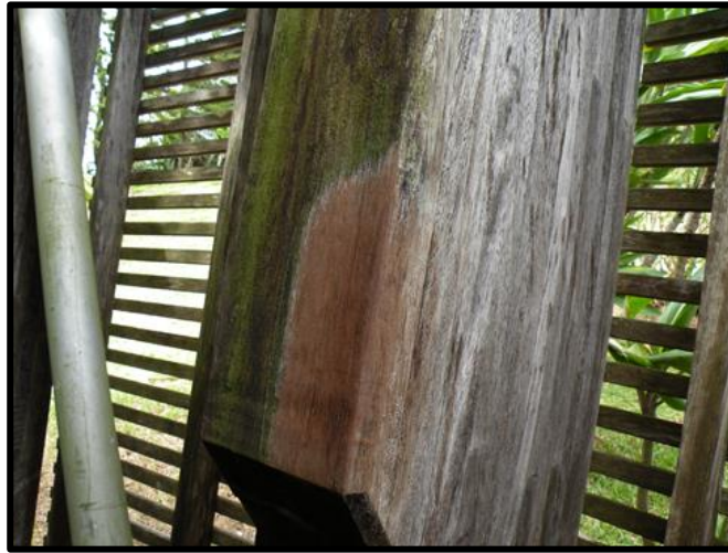
Figure 4.7. Biological growth and weathered patina, both of which can be removed through cleaning, as shown here.
