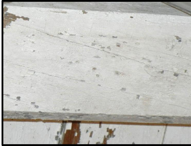
Figure 2.8. Slope of grain visible through the painted surface of a beam.
