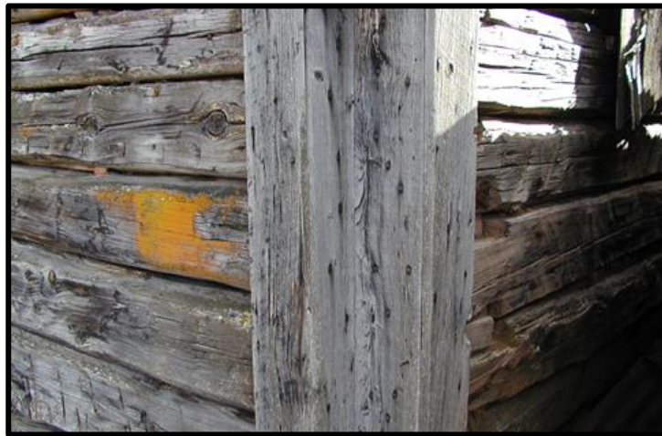
Figure 4.5. Lichens on the surface of a log structure.
