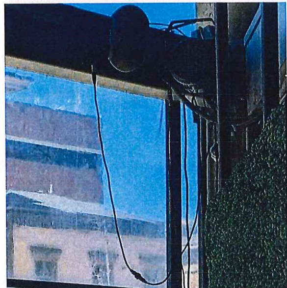
Extension cords laying everywhere and used to power the wall mounted heaters or lights
