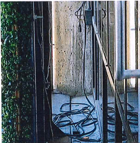
Extension cords laying everywhere and used to power the wall mounted heaters or lights
