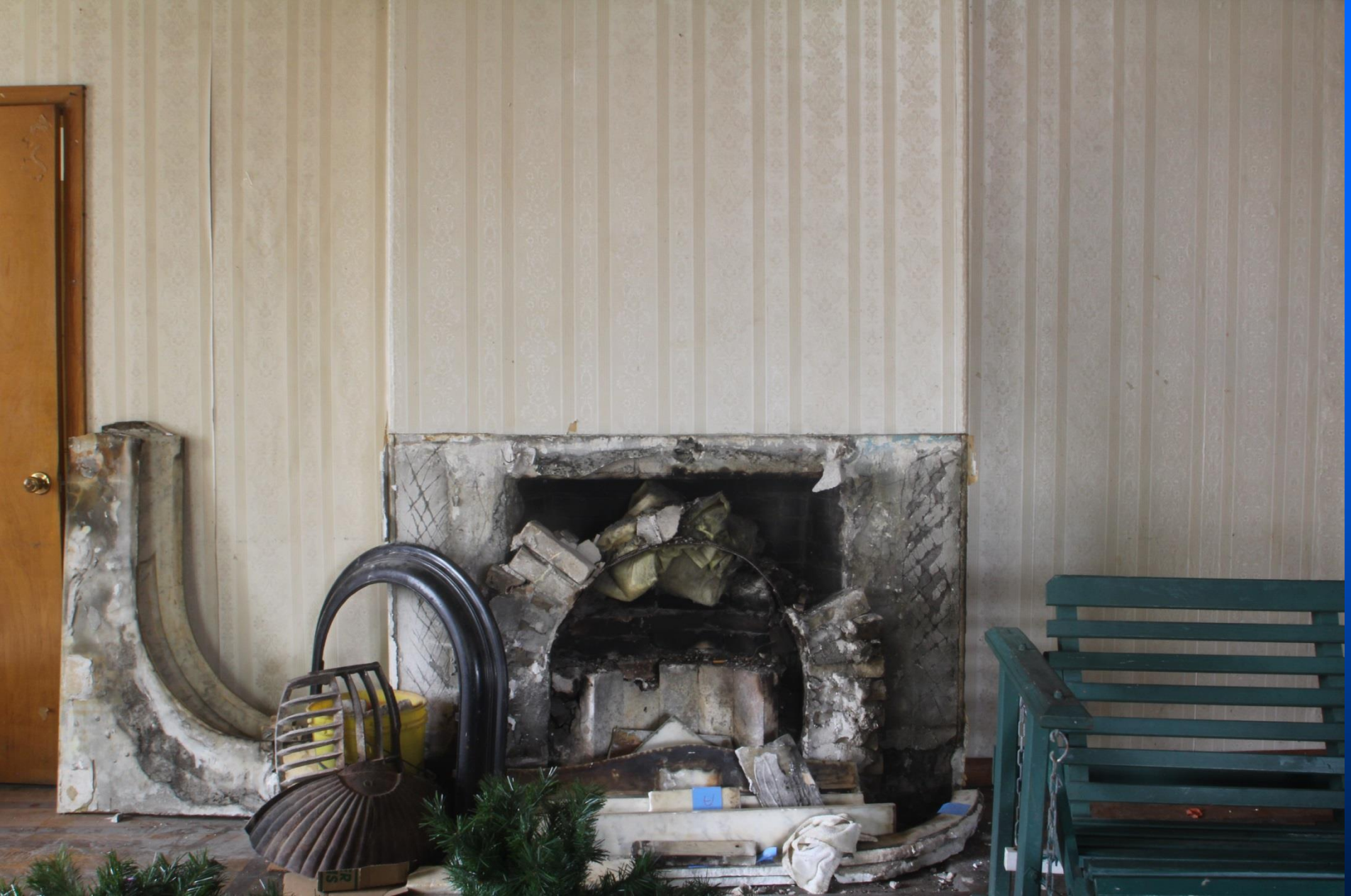
NORTH PARLOR FIREPLACE
