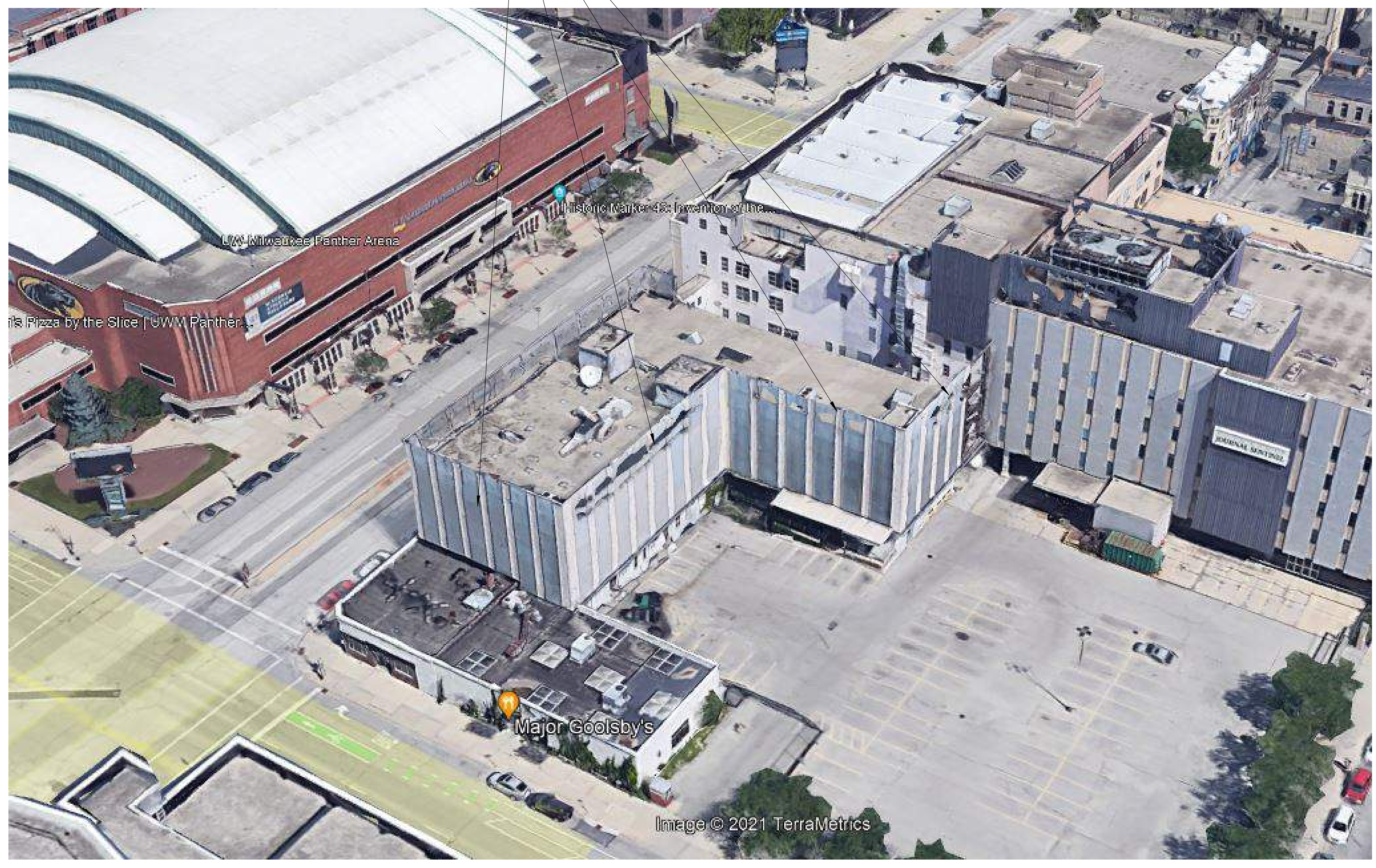
CURRENT SOUTH AERIAL
