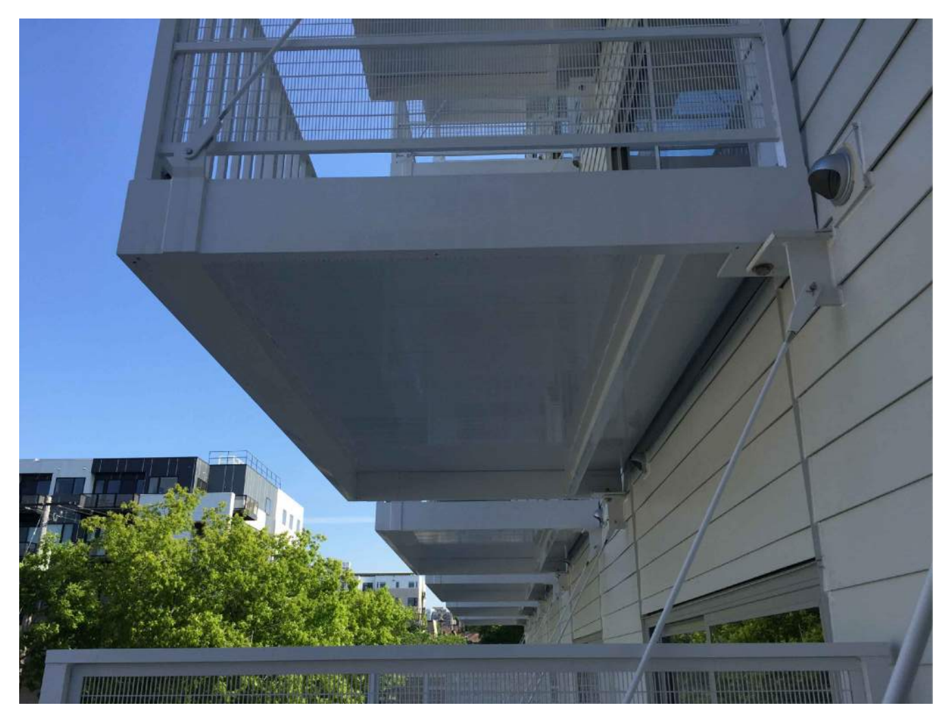
3 PRE-FABRICATED, PRE-FINISHED ALUMINUM BALCONIES DETAIL
