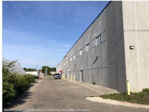
SOUTH DRIVE LOOKING WEST (PRINCIPAL BUILDING ON RIGHT)
