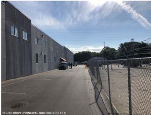
SOUTH DRIVE (PRINCIPAL BUILDING ON LEFT)
