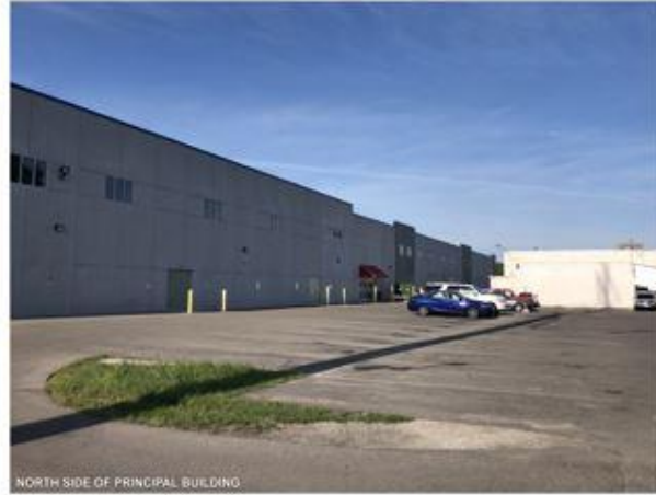
NORTH SIDE OF PRINCIPAL BUILDING
