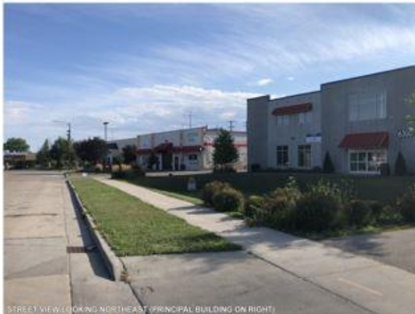
STREET VIEW LOOKING NORTHEAST (PRINCIPAL BUILDING ON RIGHT)
