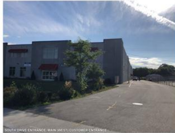
SOUTH DRIVE ENTRANCE, MAIN (WEST) CUSTOMER ENTRANCE
