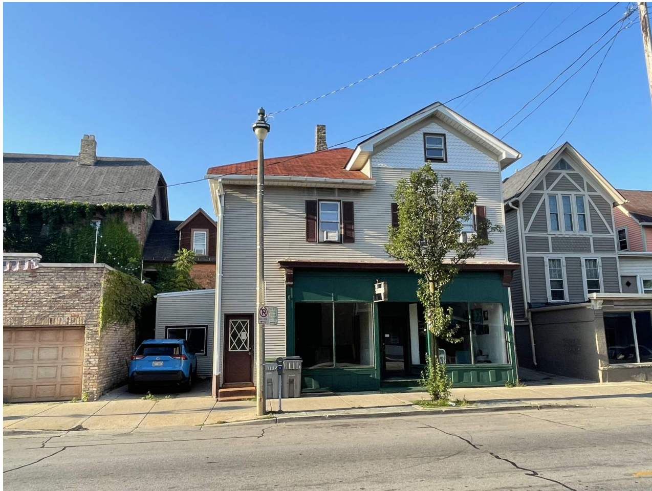
Existing Condition Photograph
