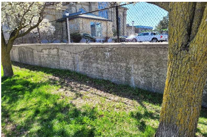
Existing N concrete retaining wall at along W. Lincoln Ave. to be clad in stone full height (approx. 86LF x 5FT tall) with stone cap.
