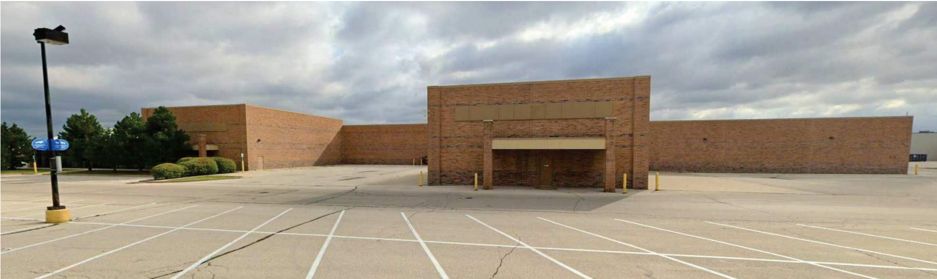
WEST SIDE OF EXISTING BUILDING
