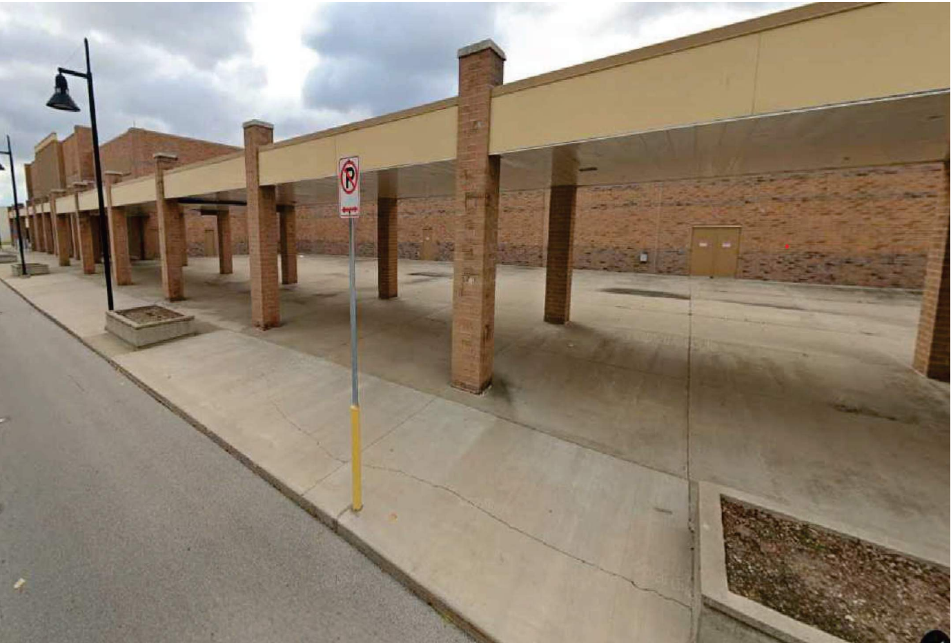
NORTH FACE OF BUILDING - COLONNADE
