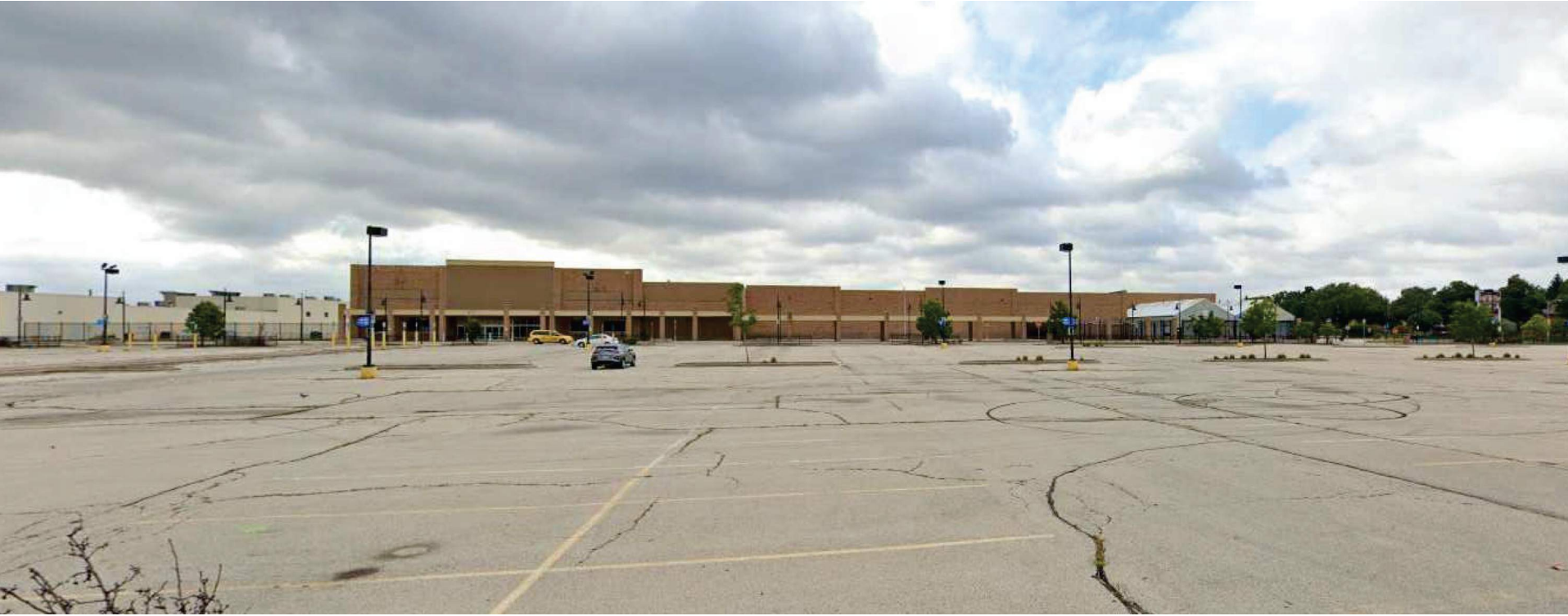
NORTH FACE OF EXISTING BUILDING
