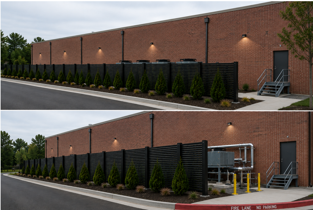
EXAMPLE ENGINEERED ACOUSTIC SCREEN WALL SYSTEM
