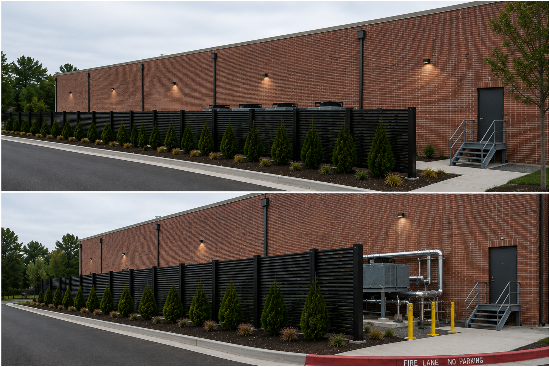
EXAMPLE OF ENGINEERED ACOUSTIC SCREENING WALL SYSTEM
