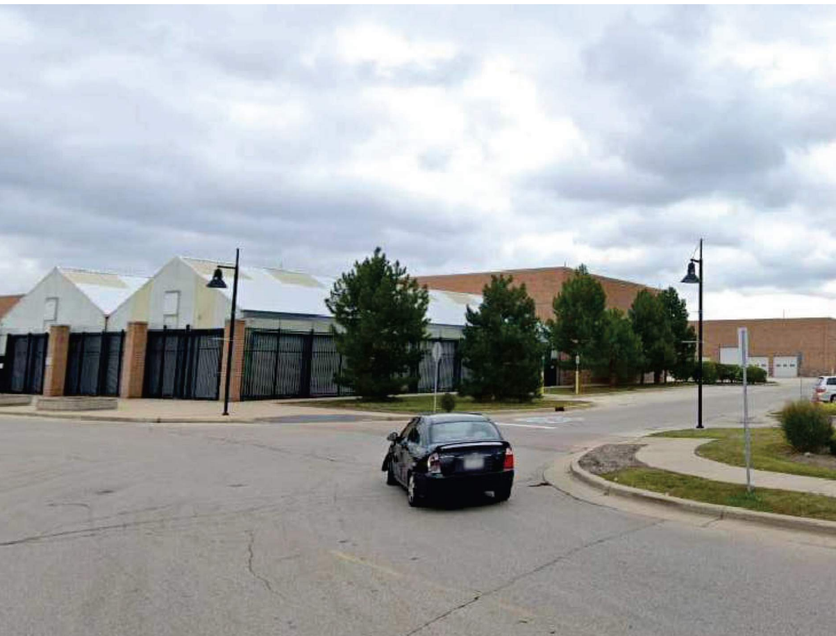
NORTHWEST SIDE OF BUILDING - EXISTING GREENHOUSES
