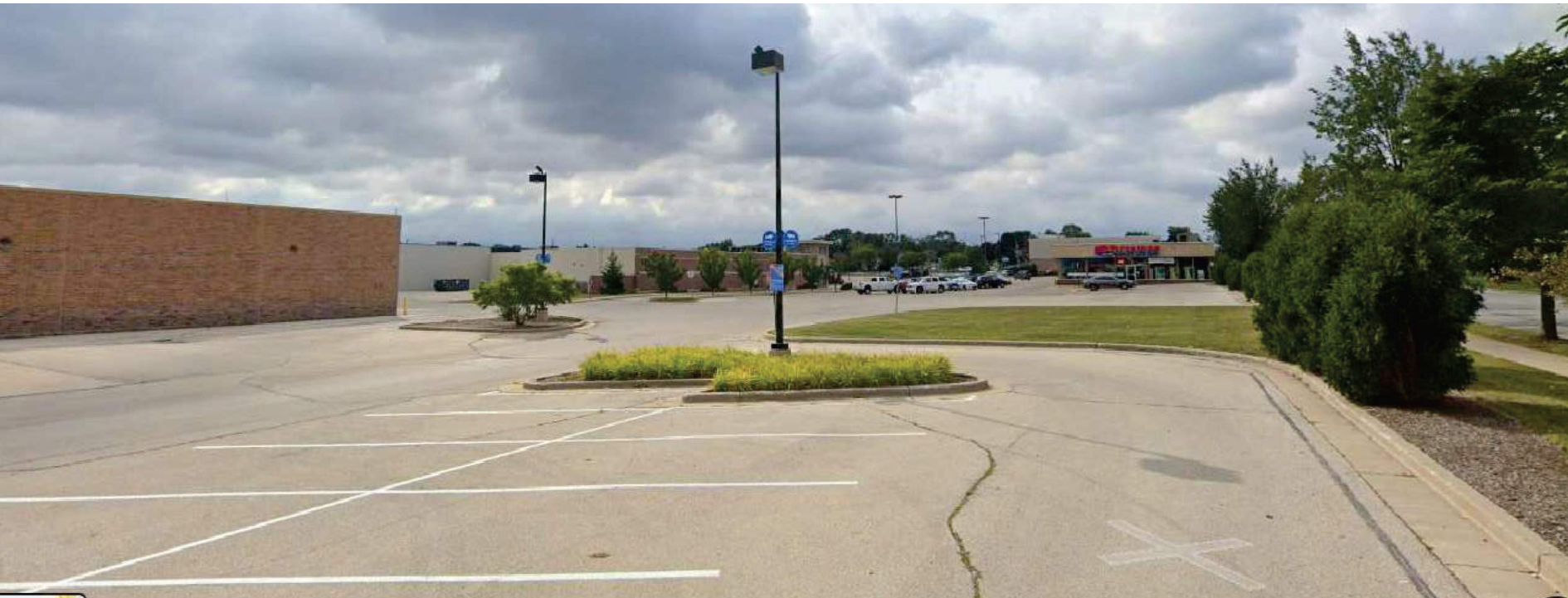
SOUTHWEST CORNER OF EXISTING BUILDING
