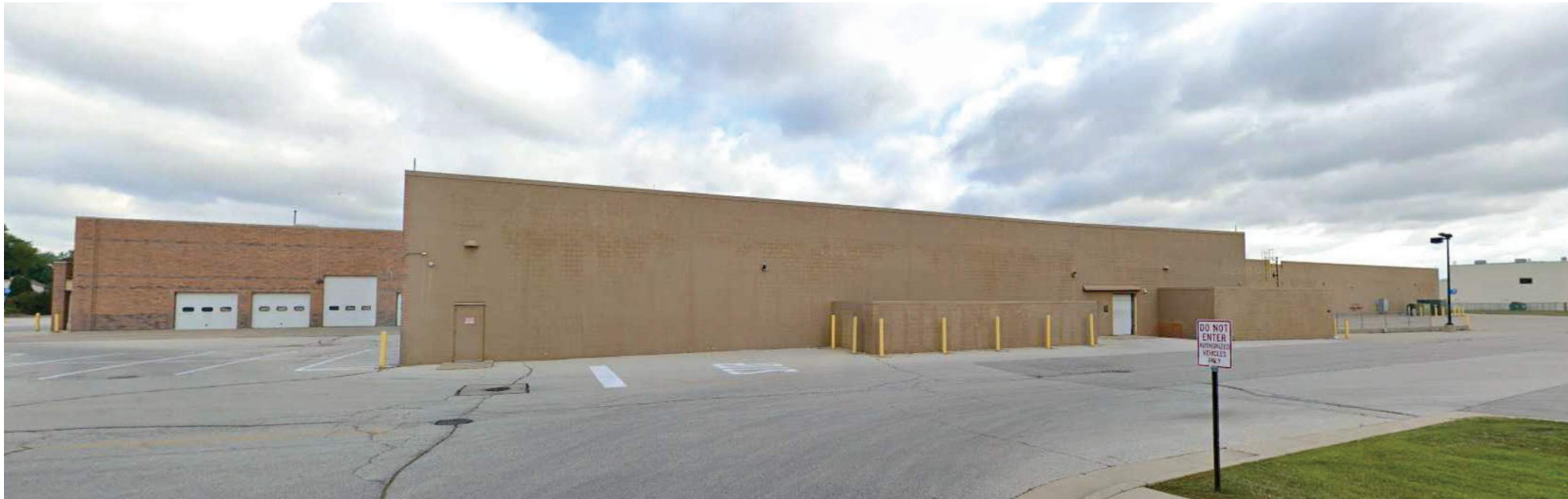
SOUTH SIDE OF EXISTING BUILDING
