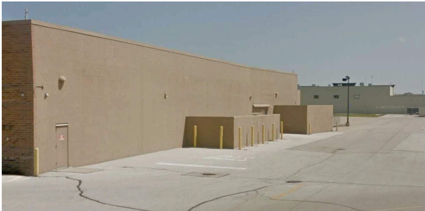
SOUTH SIDE OF EXISTING BUILDING
