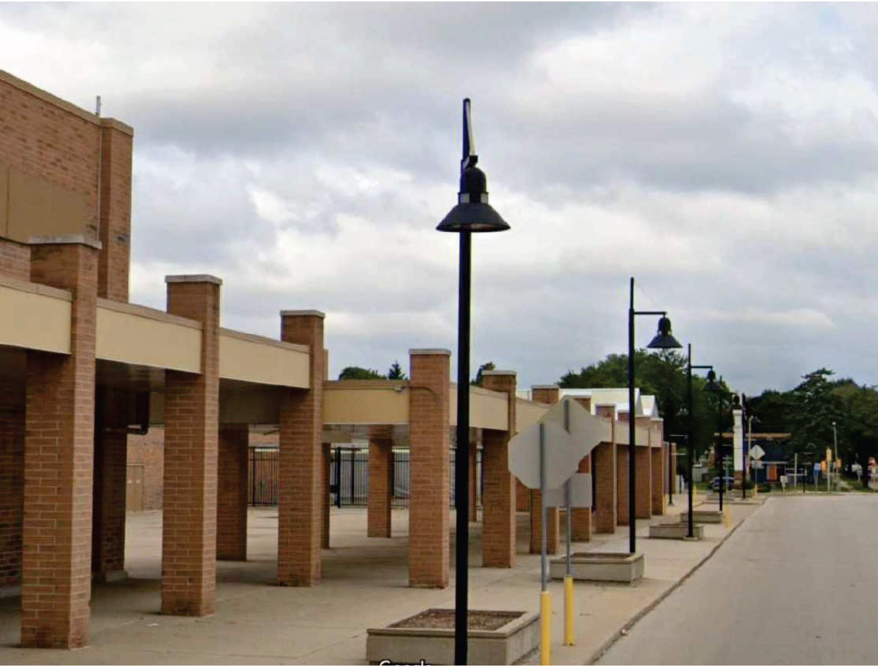
NORTH SIDE OF BUILDING LOOKING WEST
