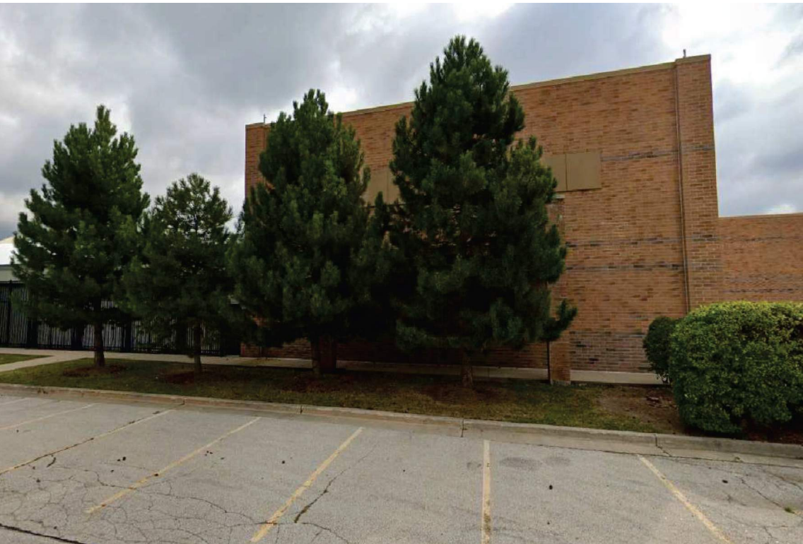
WEST SIDE OF EXISTING BUILDING
