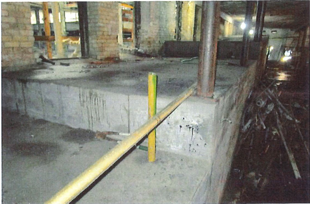
East Block, Building 1B S – Existing stepped tunnel cap (to be removed)
