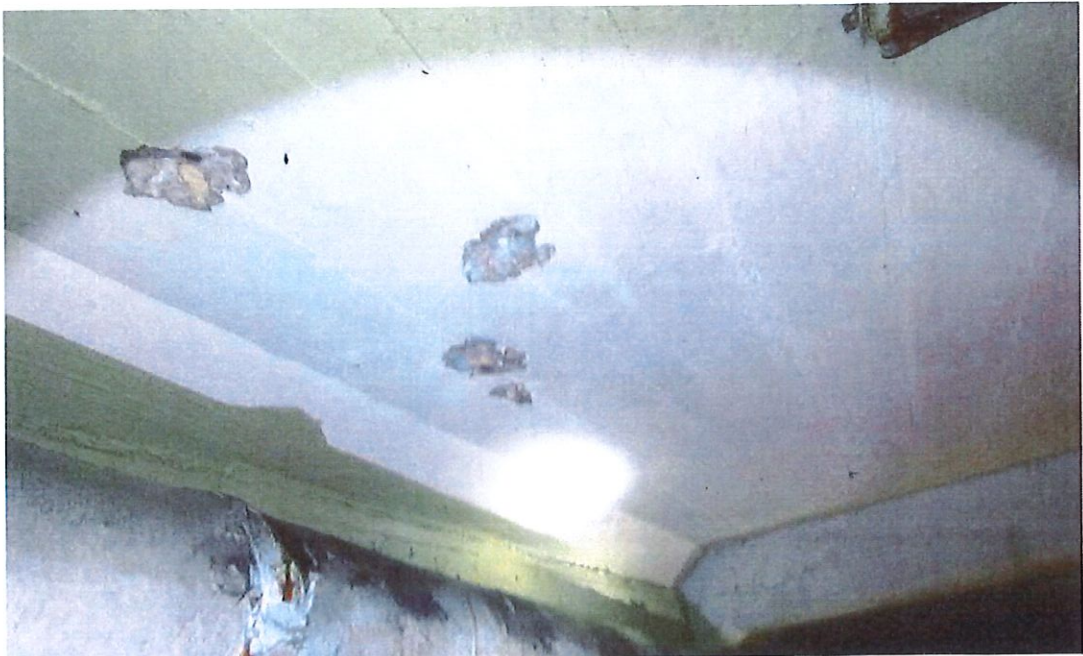
Minor spalling at ceiling
