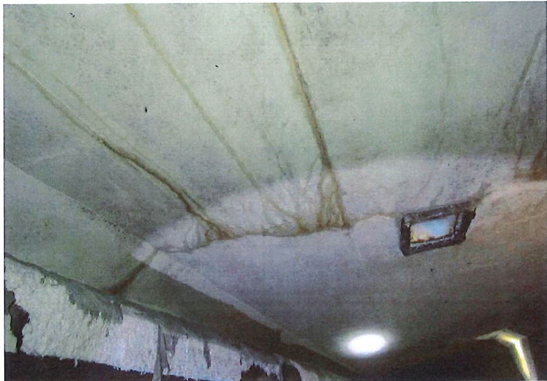
Crack in ceiling, with rust staining
