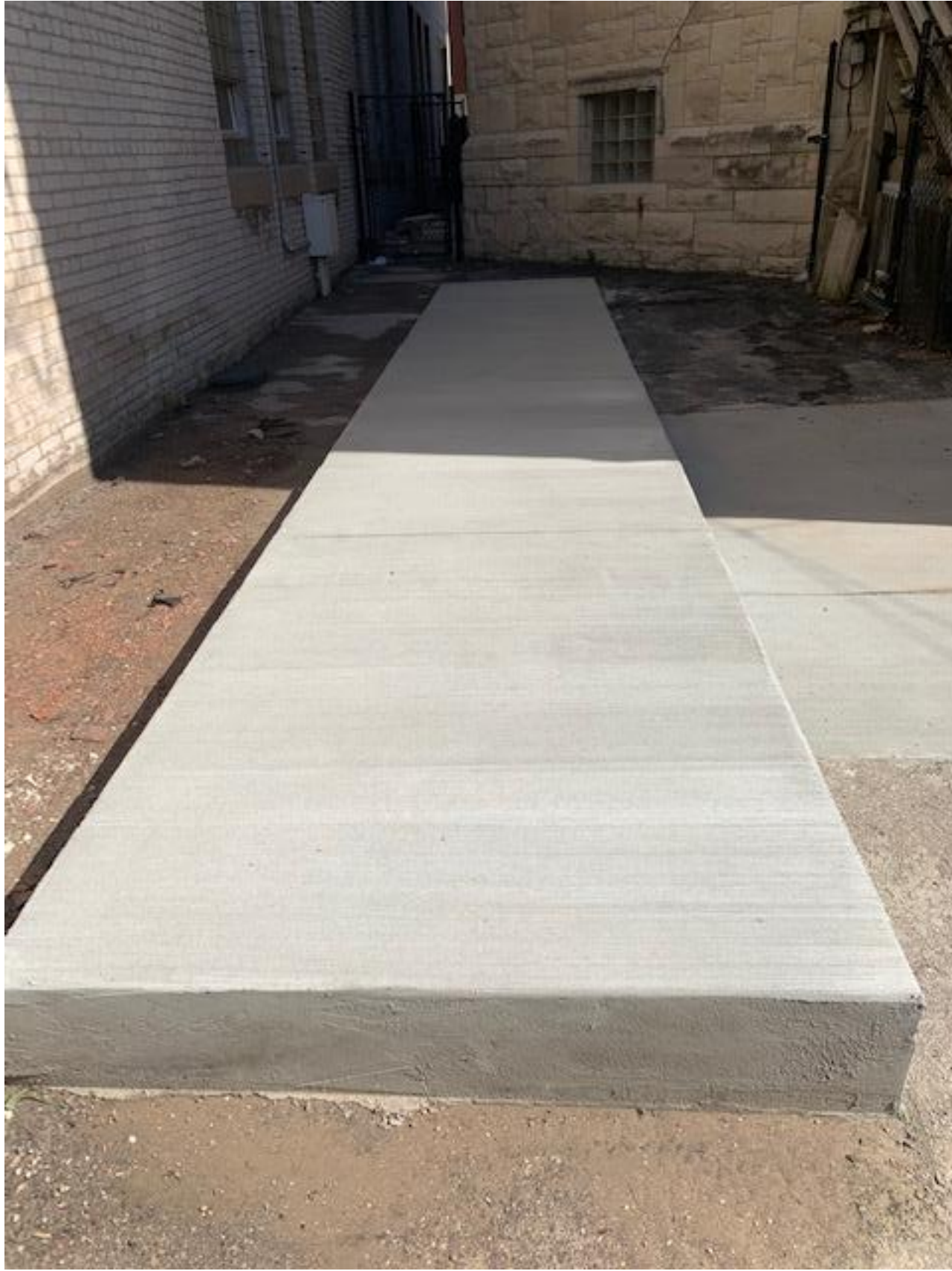
Images of the site and concrete platform that will house the three outdoor condenser units
