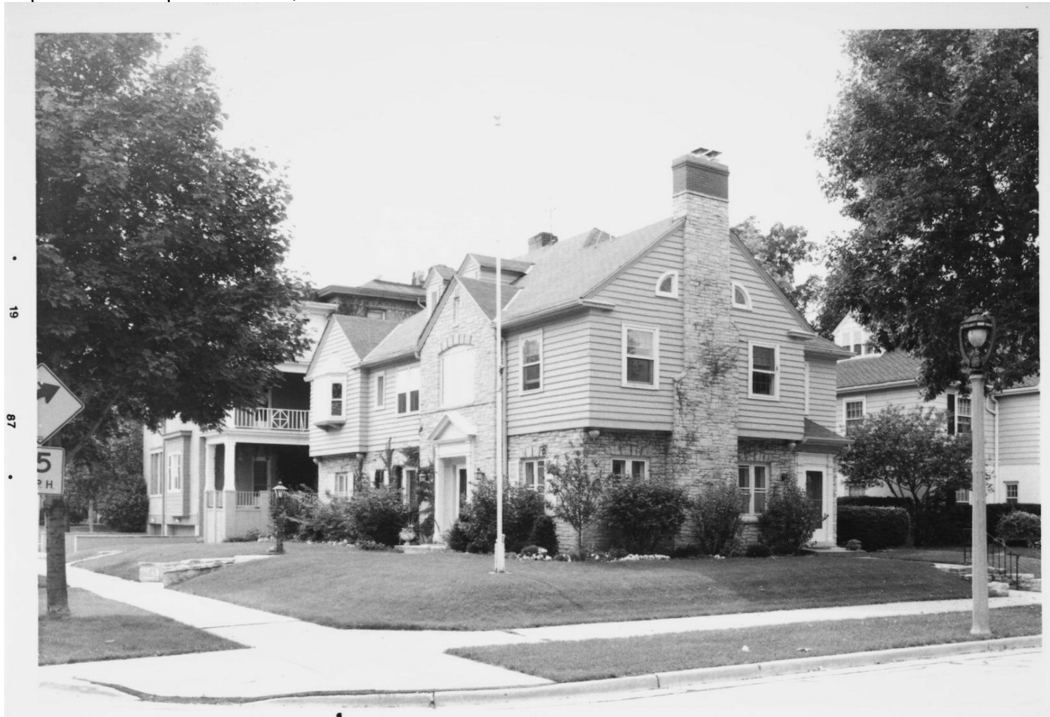
Photo from 1987. Notice mitred inside and outside corners of second floor siding.
