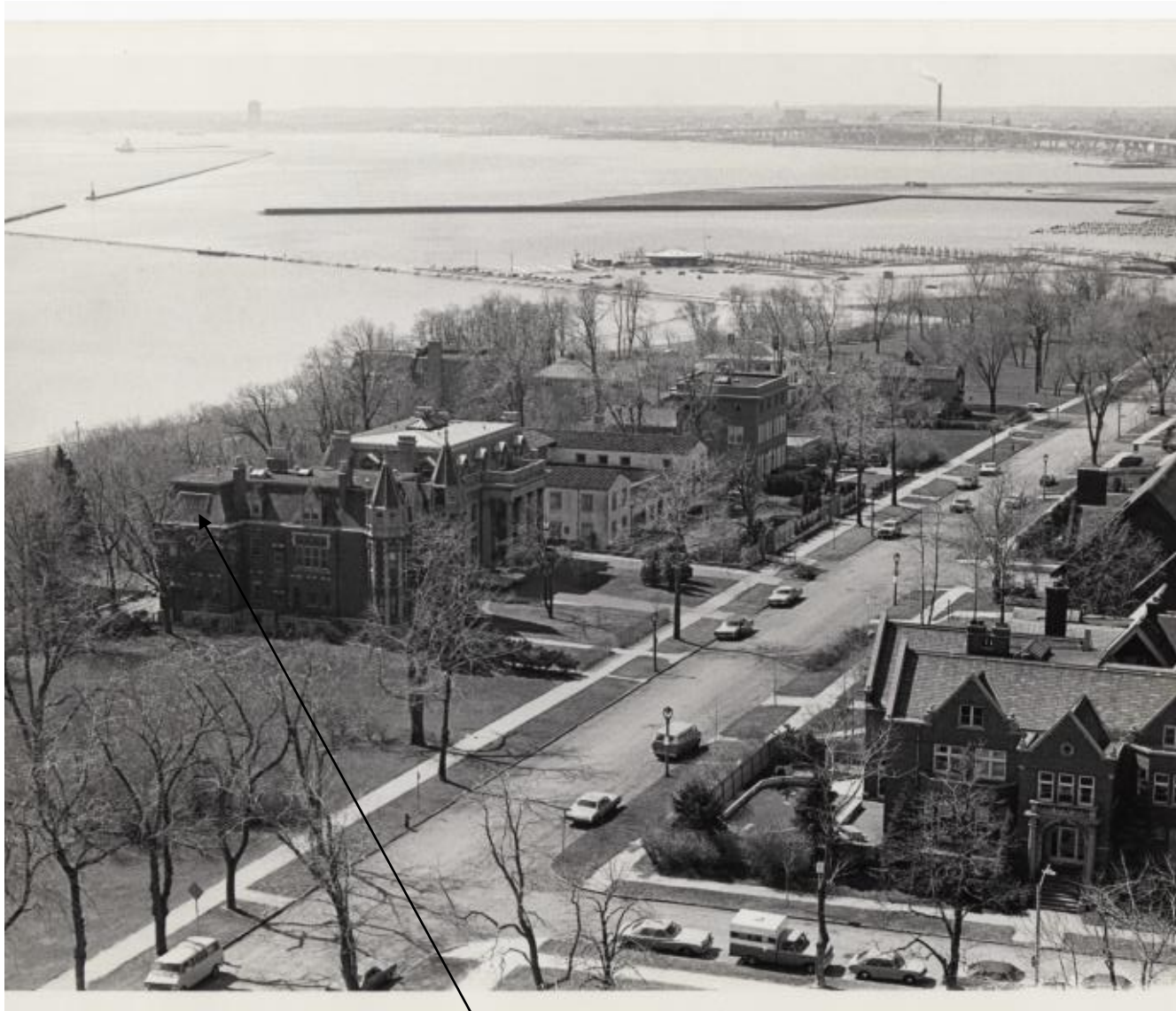
Photo taken after the Otto Herbert Falk House and the Frank R. Falk House (to the left or north) were demolished in 1968. Skylight is present on house.
