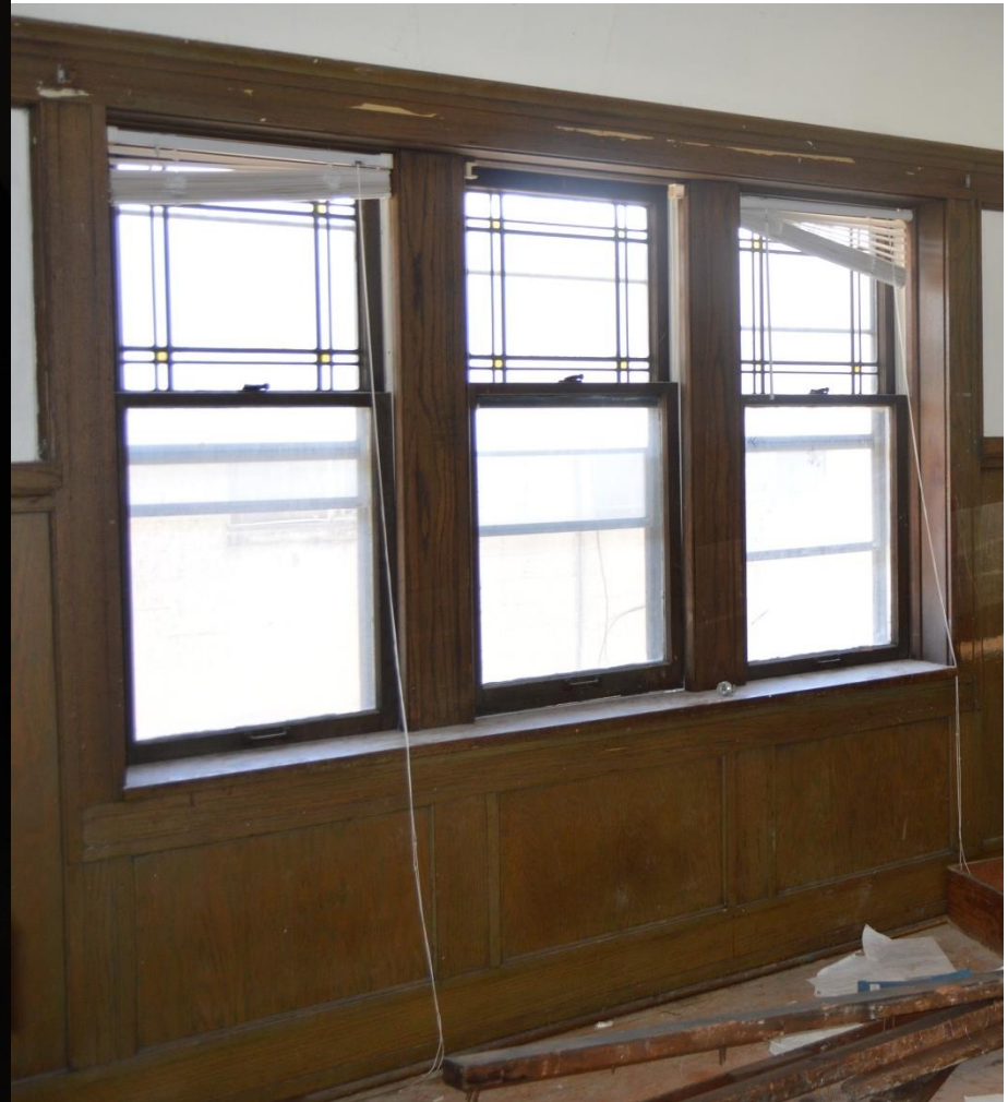
Typical leaded glass window with the small stained glass components. Rectangular sash come in two different sizes. Round-top sash exist only in the one size shown.
