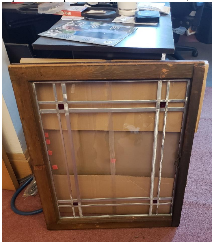
Approved replicated window sash with non-lead caming.
