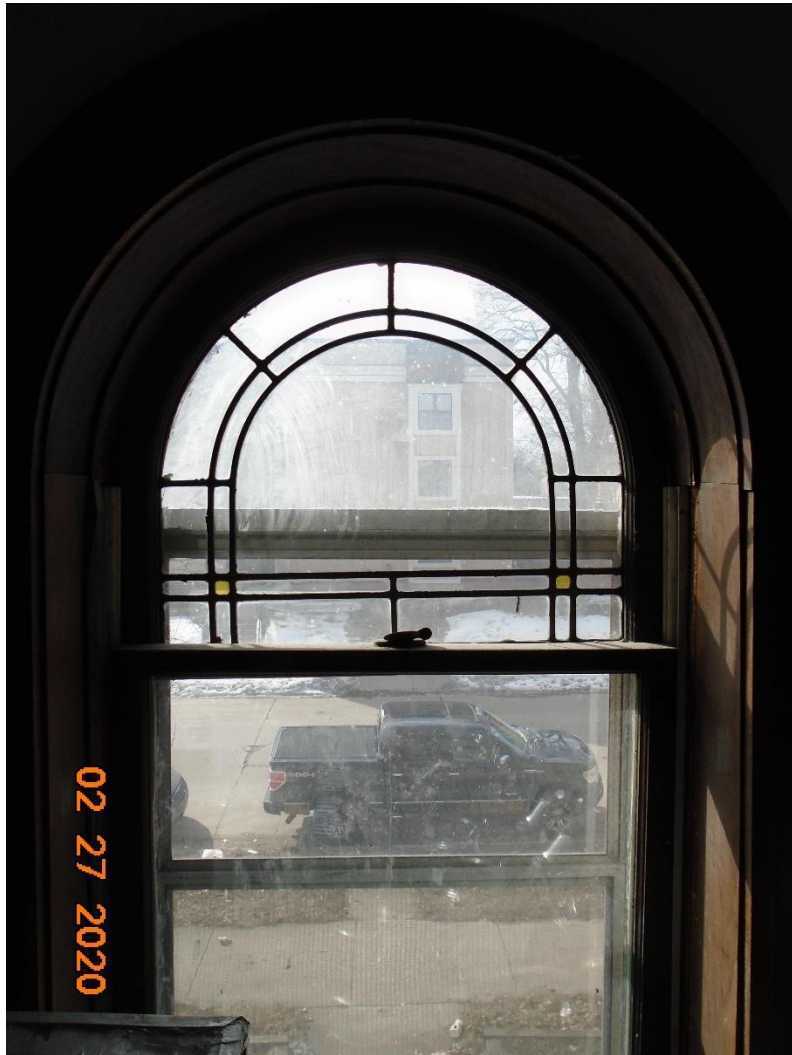
Typical leaded glass window with the small stained glass components. Rectangular sash come in two different sizes. Round-top sash exist only in the one size shown.
