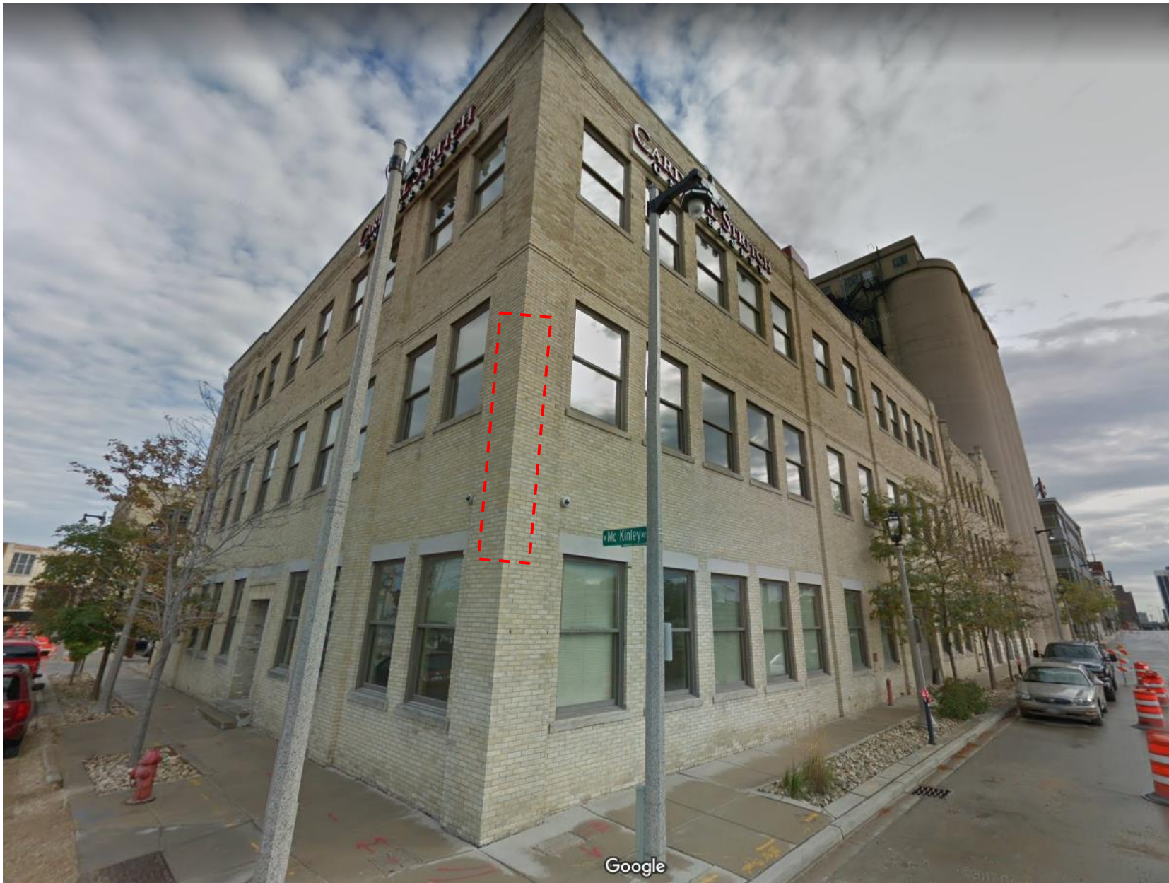
Building appearance ca. 2017 Looking SW (at NE Corner) Sign to be installed in region indicated in red
