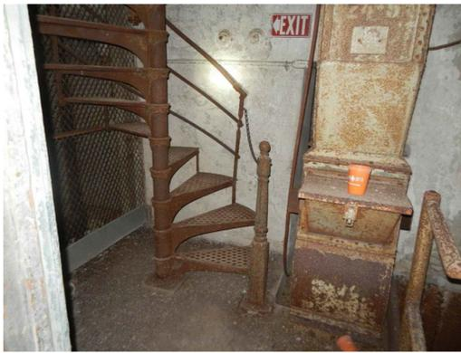
(K1) METAL SPIRAL STAIRS TO BE REPURPOSE AT THE ATRIUM ON THE NORTH SIDE OF THE PROPOSED NORTH PASSENGER ELEVATOR.
