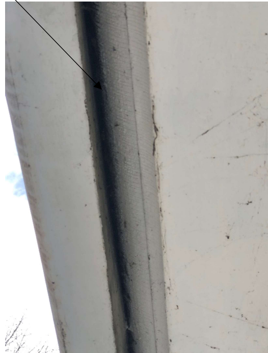
The existing fascia is inverted
