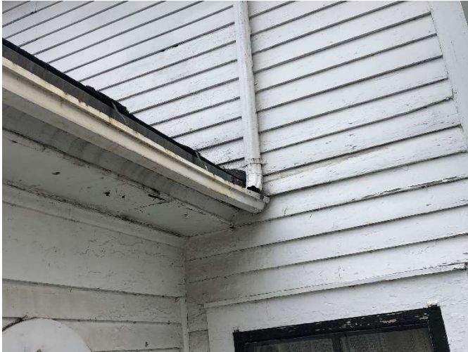
The existing fascia is inverted
