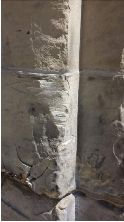
Photos 17-19 – Typical conditions of Cleveland sandstone corners, pilaster base.
