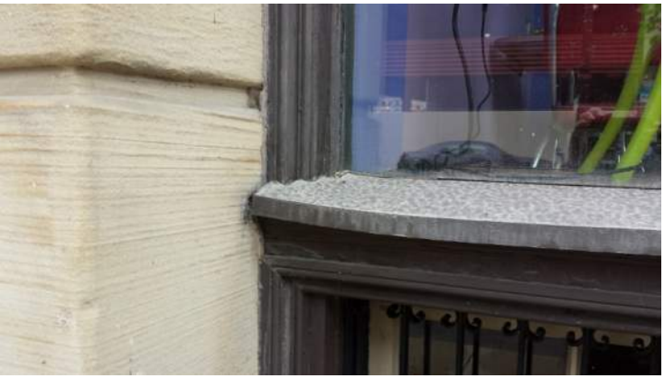
Photo 15, 16 – Typical condition of replacement sill material at first floor windows.
