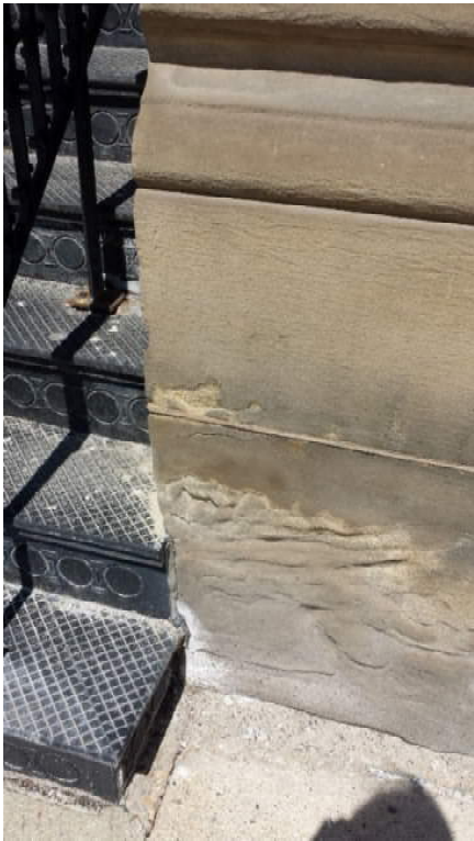
Photos 20,-22 – Southern elevation, typical conditions of Cleveland sandstone base with presence of spalling, efflorescent salts..
