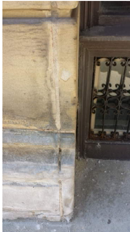
Photos 20,-22 – Southern elevation, typical conditions of Cleveland sandstone base with presence of spalling, efflorescent salts..
