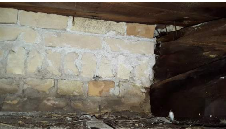
Photo 9 - Interior cornice wood-support structure – dry.
