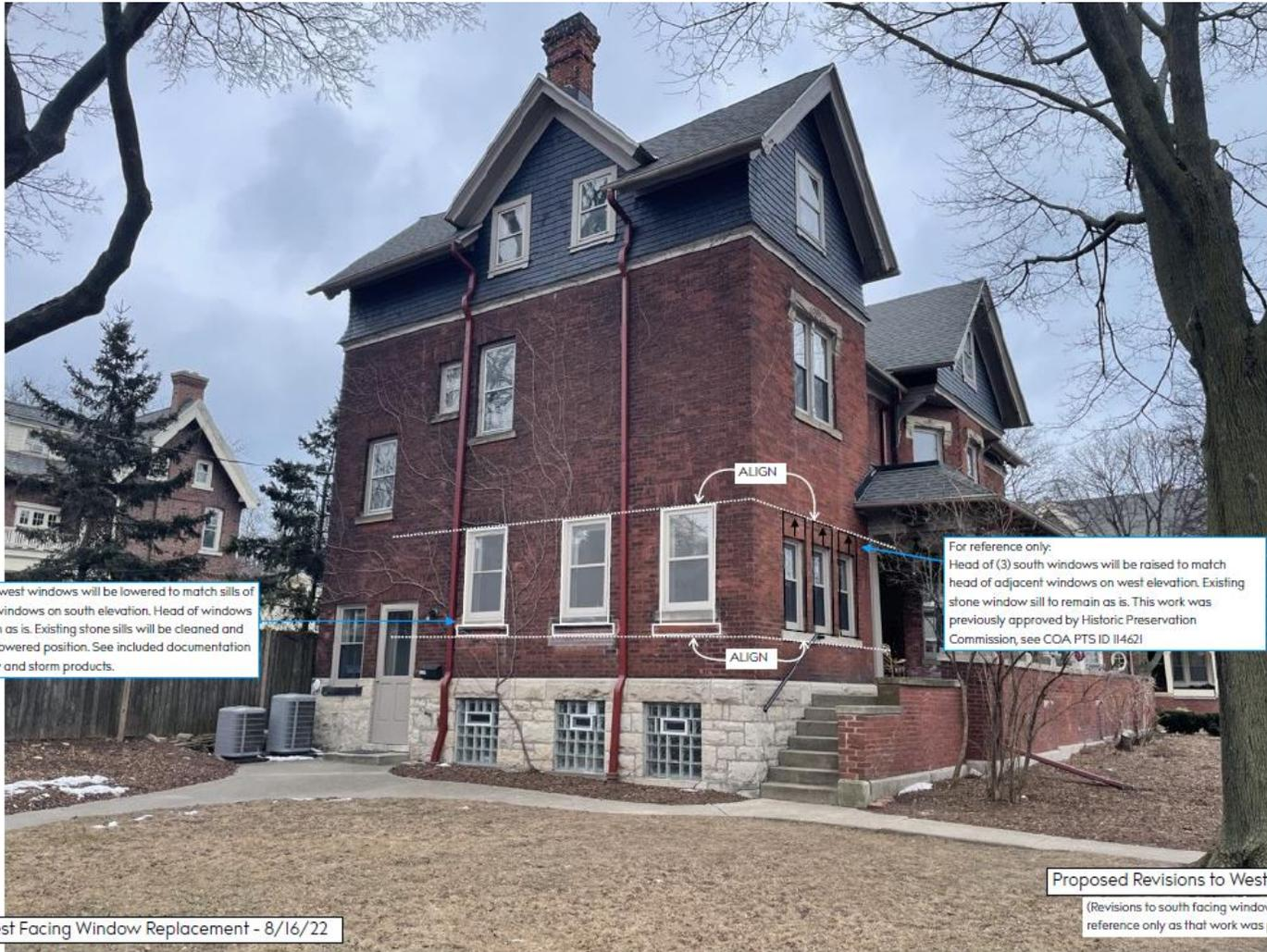
Sills of (3) west windows will be lowered to match sills of adjacent windows on south elevation. Head of windows will remain as is. Existing stone sills will be cleaned and reused in lowered position. See included documentation of window and storm products.
