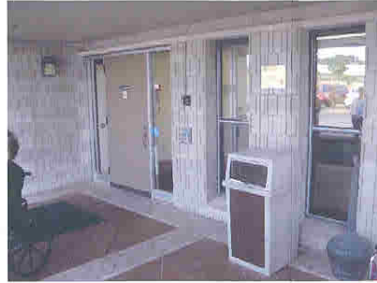
EXISTING MAIN ENTRANCE DOOR AT PROPOSED VESTIBULE
