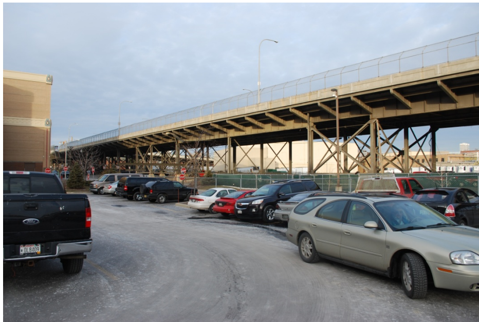
North East View from Parking Structure Site
