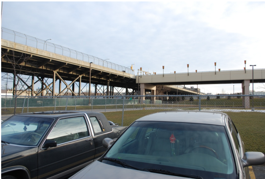
South East View from Parking Structure Site
