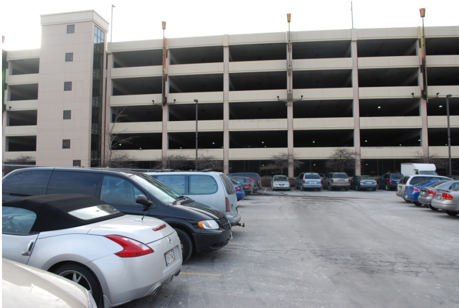
West View from Parking Structure Site
