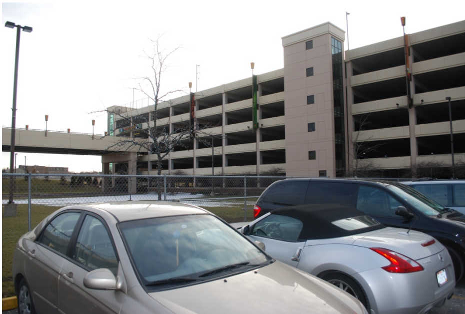
South West View from Parking Structure Site
