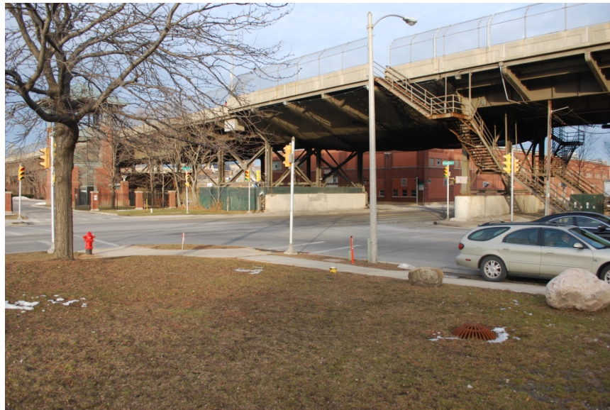
North East View from Hotel Site
