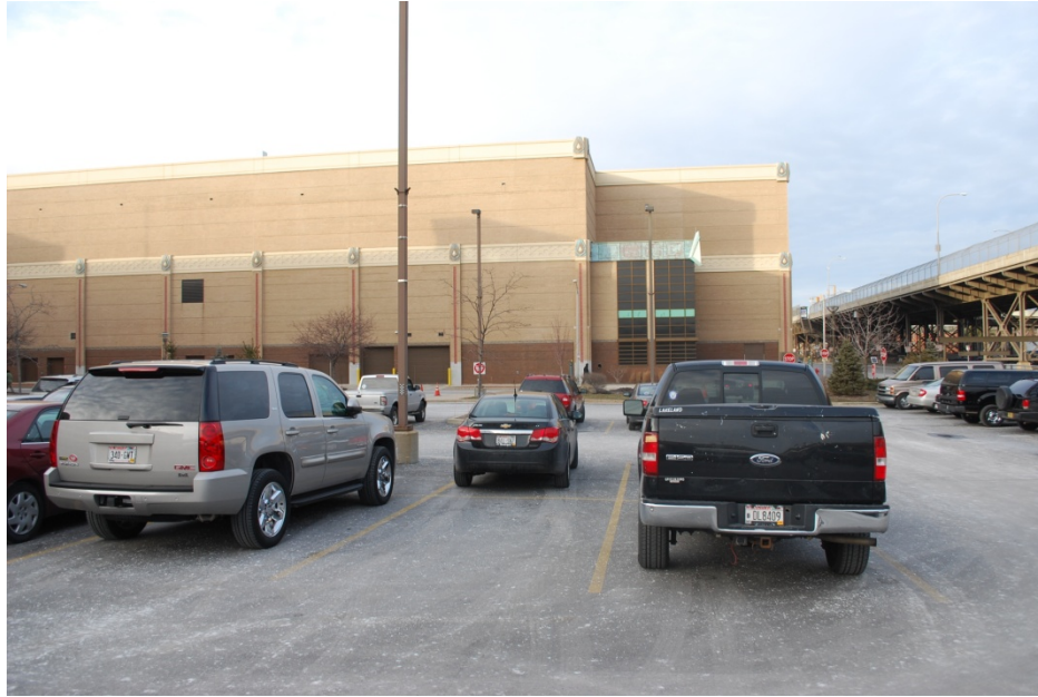
North View from Parking Structure Site
