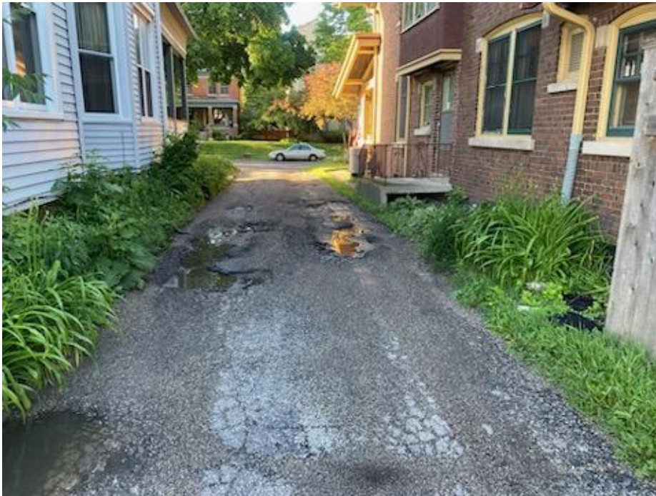
Condition of existing asphalt driveway.
