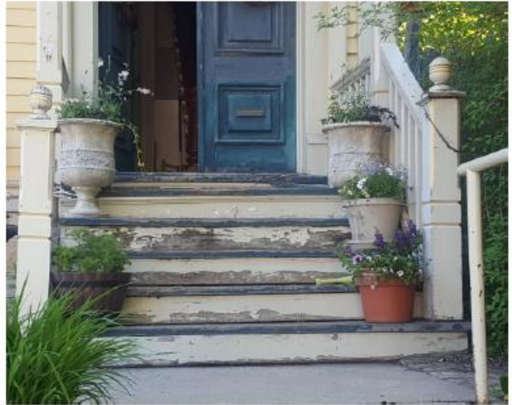
existing porch to be repaired (prior to house painting)
